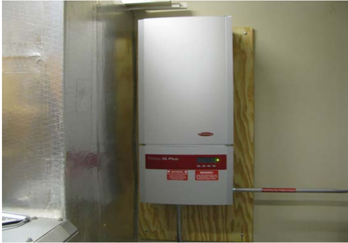
Feronius Converter located in Dining Hall Electrical Room. Last stop for the solar electricity.
