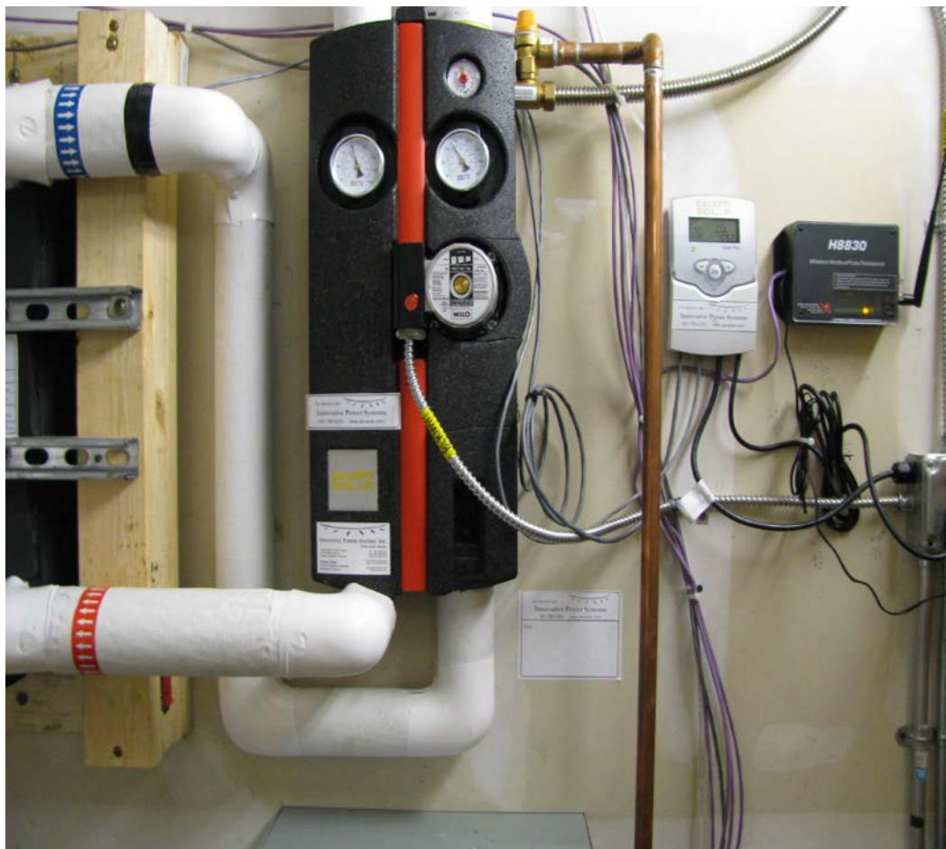
Monitoring equipment at the North Star Lodge for the Solar Hot Water.
