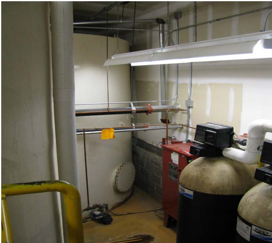
Heated water is stored in one of two 10,000 gallon hot water heaters in the North Star Lodge.
