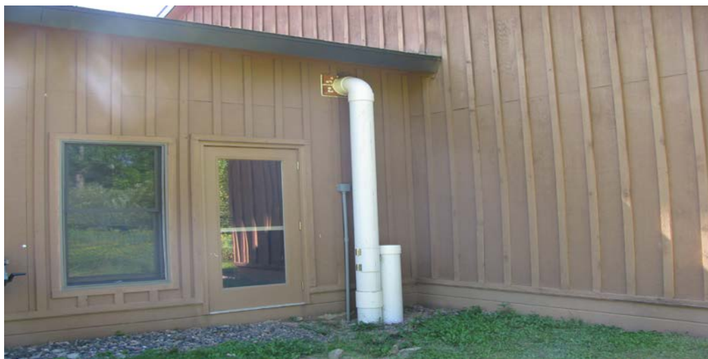
Hot water enters the North Star Lodge, line is protected by PVC pipe.
