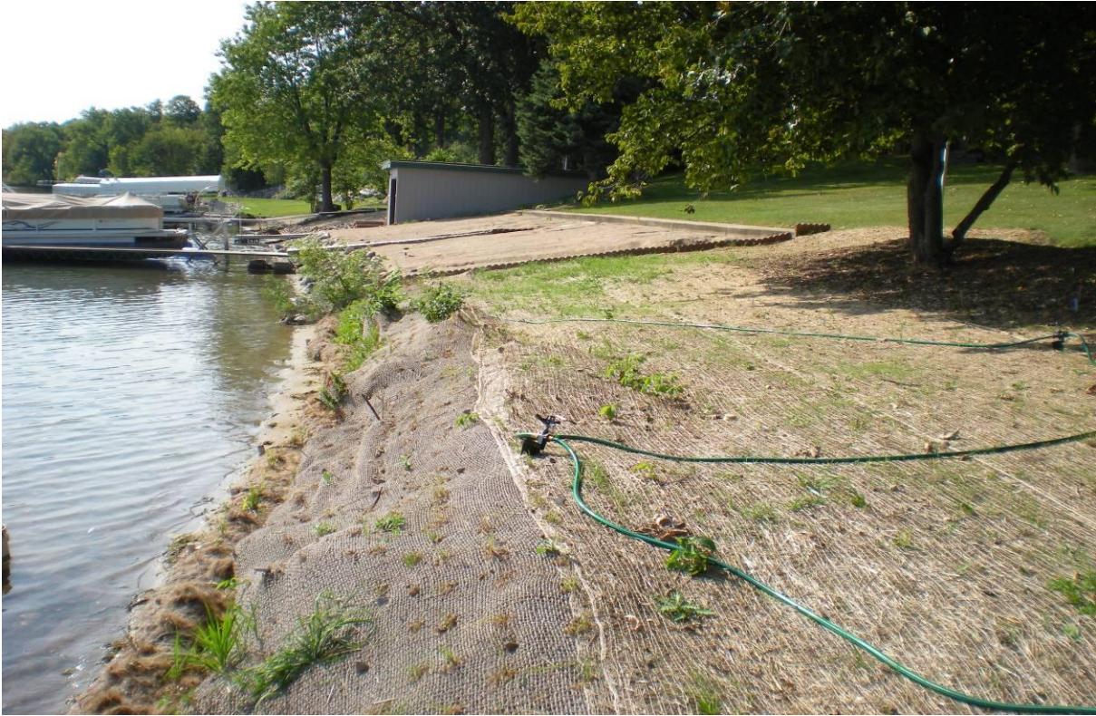
Photo 15: Sand blanket (rear) and shoreland restoration (foreground), East Otter Tail County
