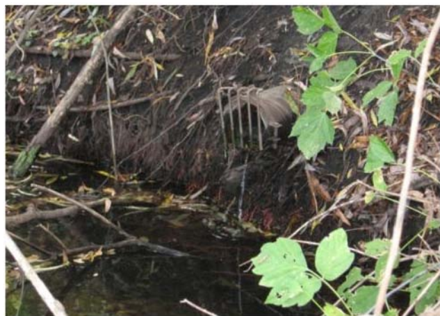
Drainage Tile Outfall along the Vermillion River
