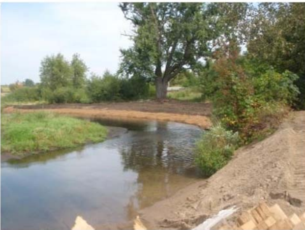
Streambank Stabilization Project
