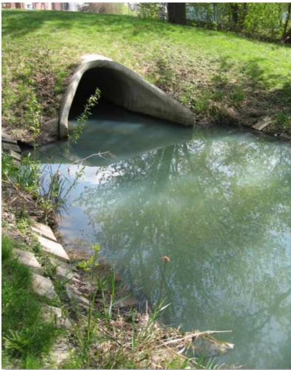
Turbidity: Stormwater Conveyed to Surface Water
