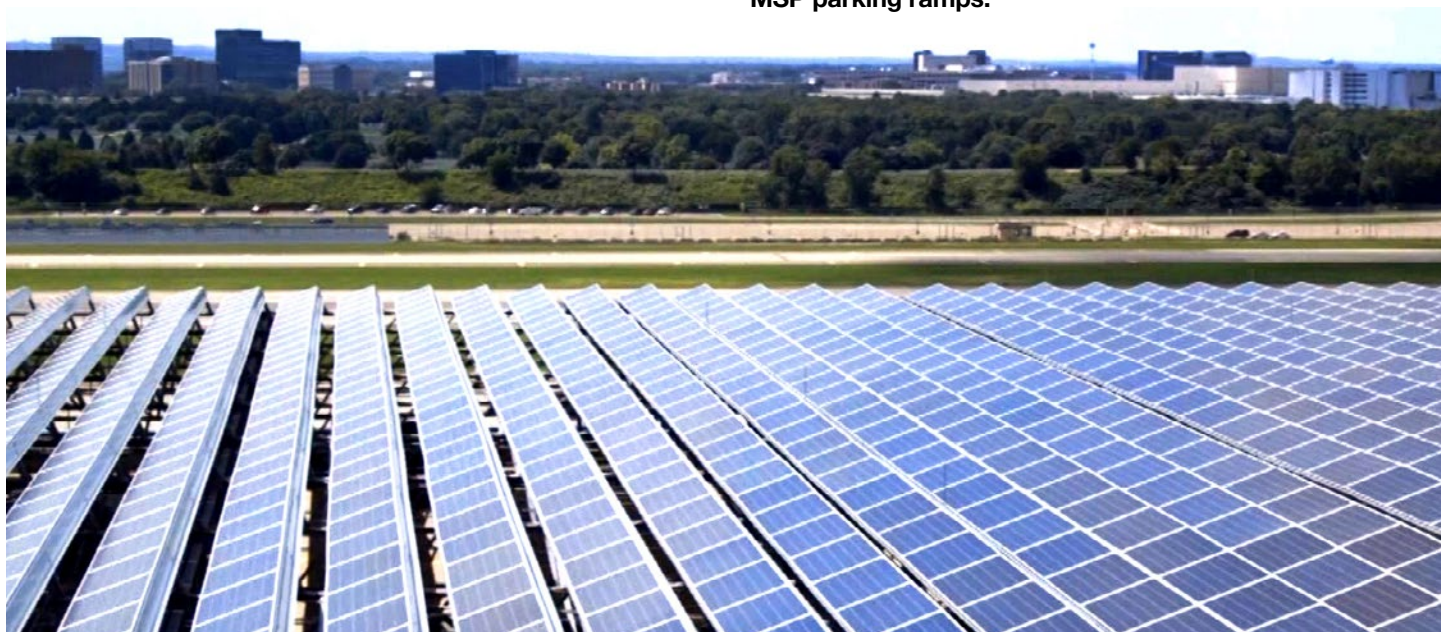
Solar Energy installation at Terminal 1-Lindbergh's parking facility.
