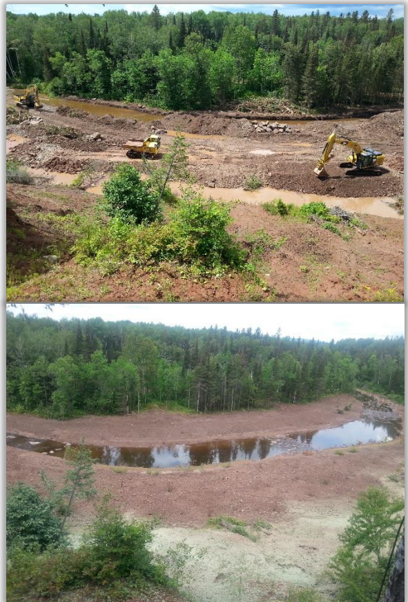
Pictured, top: Construction of the new bank. Pictured, bottom: Floodplain bench installed at the bank stabilization site on the Knife River.
