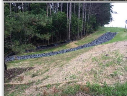
A rock lined channel was installed to stabilize a large road side gully draining directly to North Center Lake.
