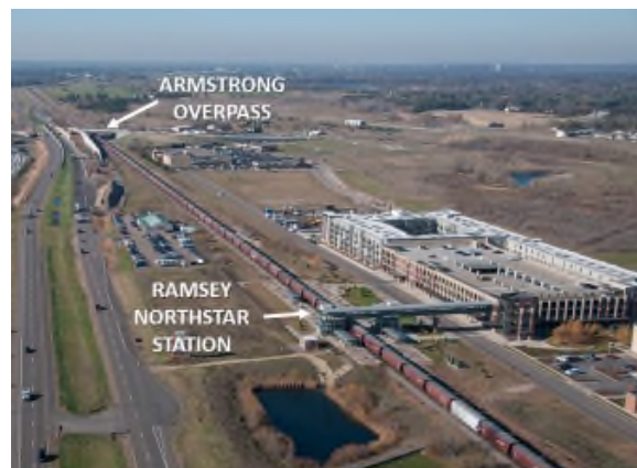
Figure 3: The Anoka County CSAH 83 Bridge over the BNSF Railroad tracks used by Northstar was completed in one construction season.
