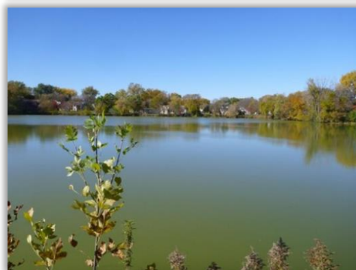
Top: The Long Lake Watershed grant includes four major projects, including the Mirror Pond Stormwater Retrofit. The pond is pictured, bottom.
