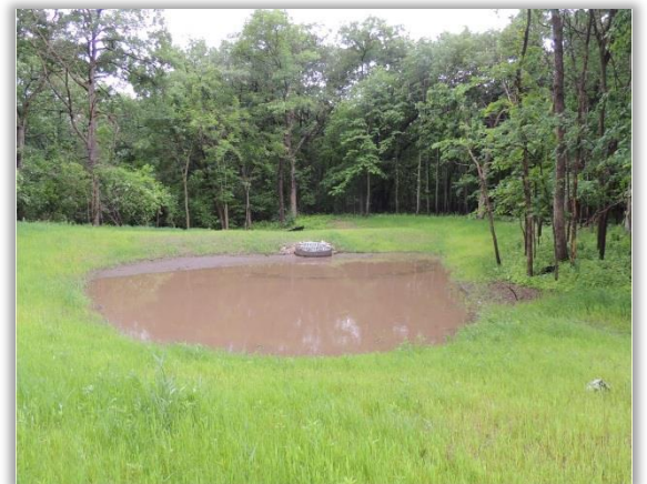
Impoundment structures like this help slow down water, minimizing erosion and helping keep sediment out of the creek.
