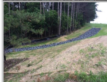
A rock lined channel was installed to stabilize a large road side gully draining directly to North Center Lake.
