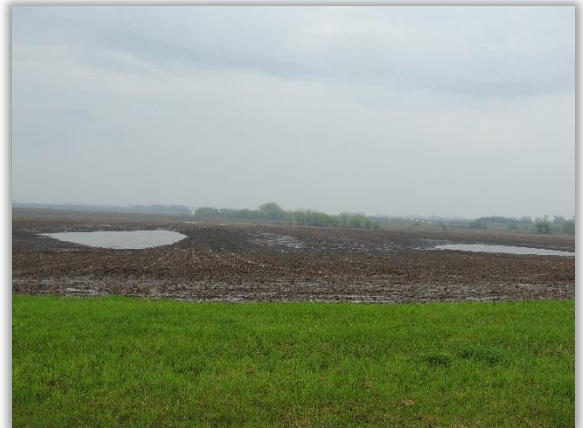
Water and sediment control basins have been installed in farm fields to help minimize flooding and keep sediment out of the creek.
