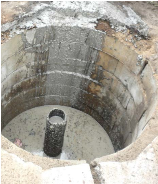
Figure 30. Well sealing project completed in Benton County
