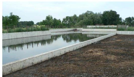
Figure 12. Manure treatment system in Stearns County.
