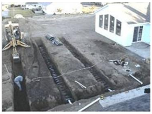
Figure 28. Typical septic system installation
