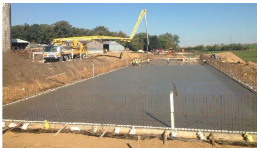
Figure 11. Typical manure storage pit under construction in Olmsted County.
