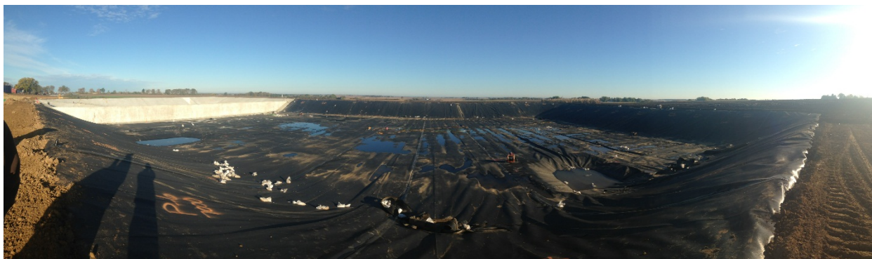
Figure 13. Installation of manure basin liner, Olmsted County.
