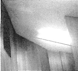
Note the air infiltration from the vent. This may be duct leakage from the attic.
