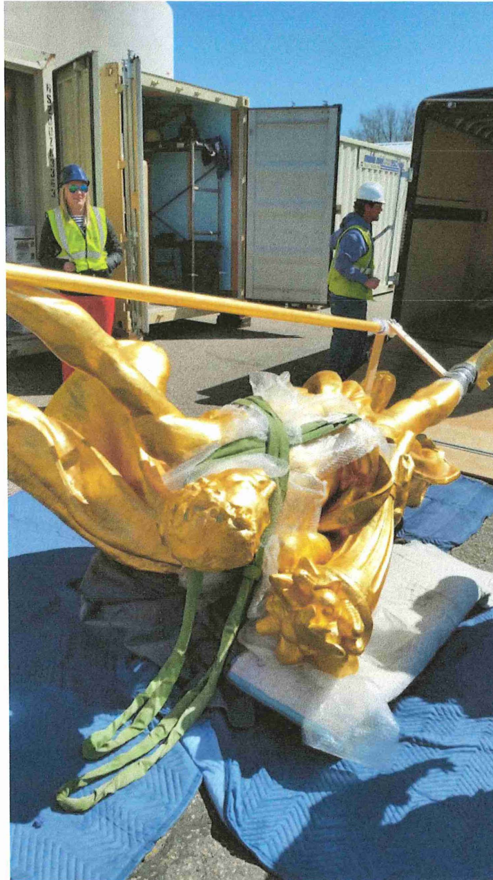
Prosperity is illustrated with rigging and braces, ready for the lift to the Quadriga . Bubble wrap protects gold surfaces during the lift.
