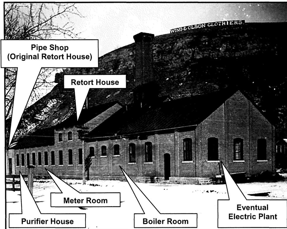
FIGURE 10. RED WING GAS AND ELECTRIC COMPANY PLANT, 1897 (MHS NEG. No. 18815)
