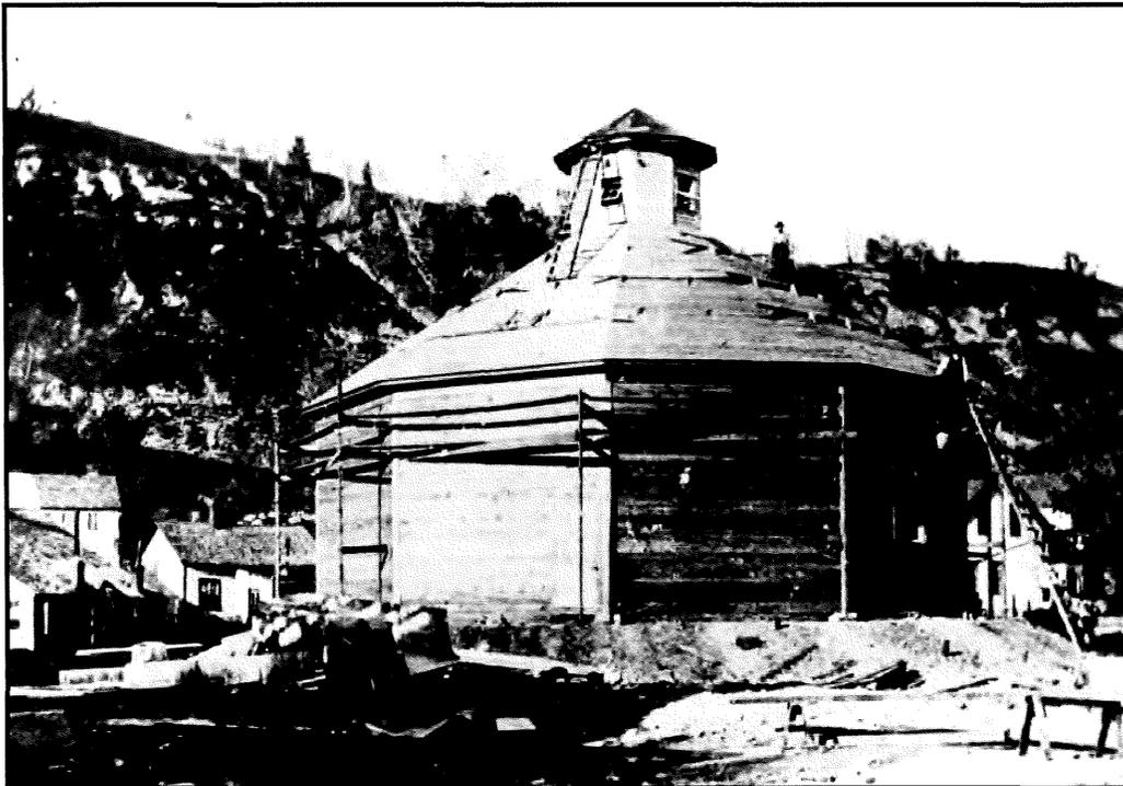
FIGURE 11. GAS HOLDER CONSTRUCTED IN 1894 AT BLUFF AND 3<sup>RD</sup> STREETS (GOODHUE COUNTY HISTORICAL SOCIETY IMAGE 1.2.4053)
