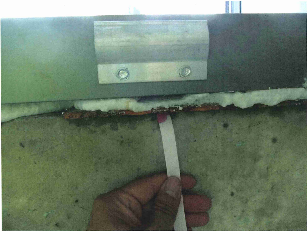
Water observed below the anchors at the sill.
