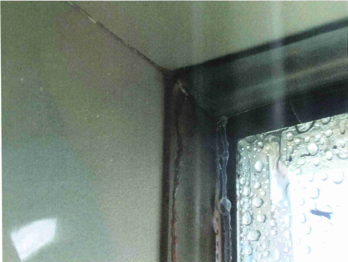
Glazing leak at the upper left corner of lower left lite.
