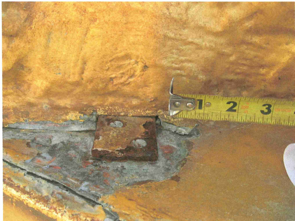
Photo 6: Photo of Leg Hold Down Strap & Bolts
