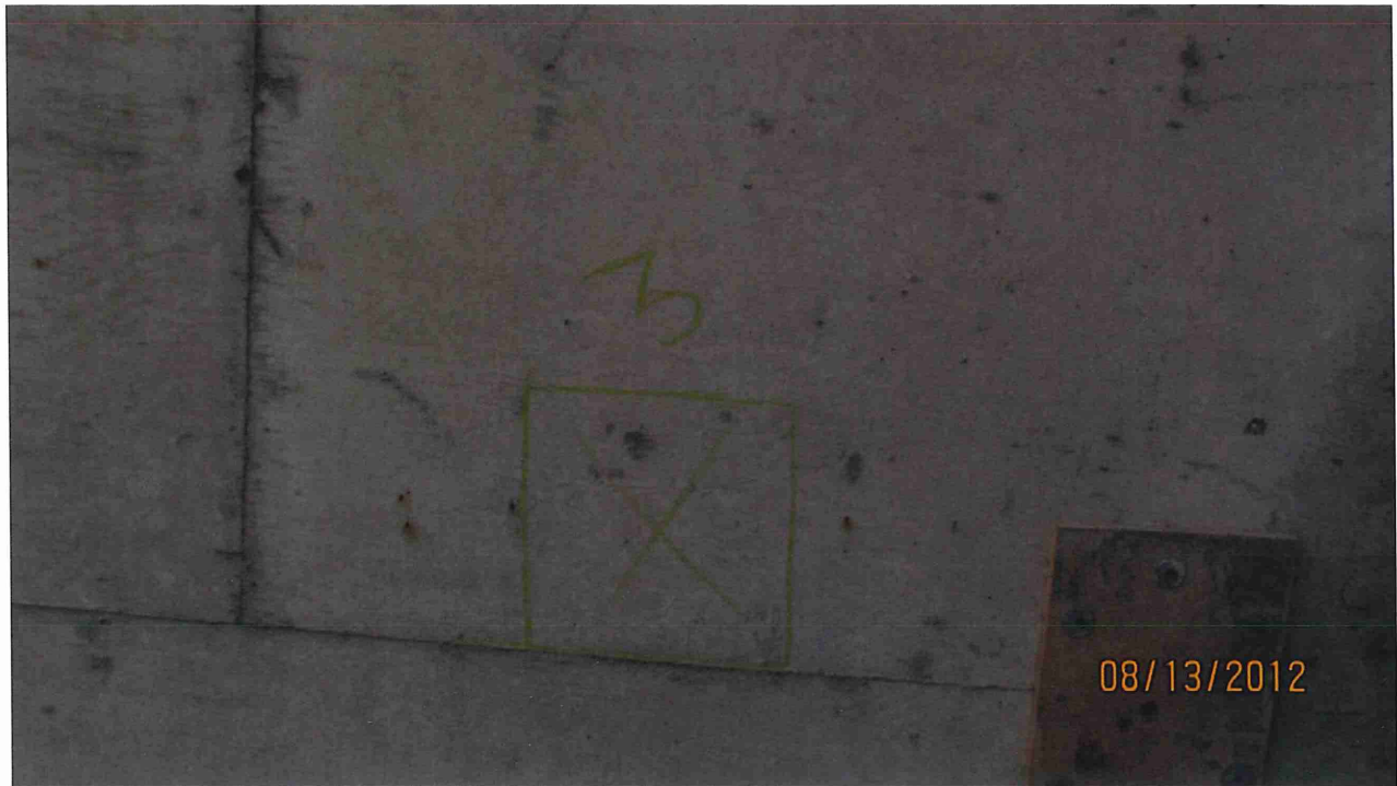
Sample # 3 is 4' North of Pier #1 and 3' west of center line. This is next to an existing patch. This was a full depth core sample that showed high chloride concentration levels,
