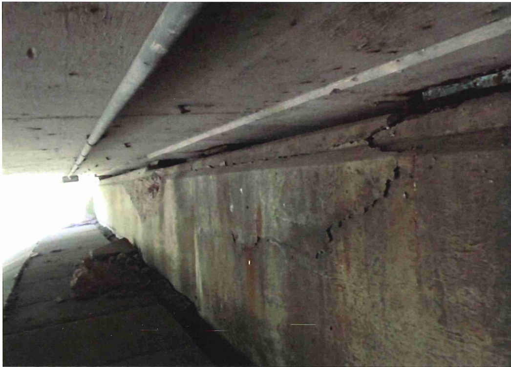
North Abutment - Additional corner spall/delamination photo.
