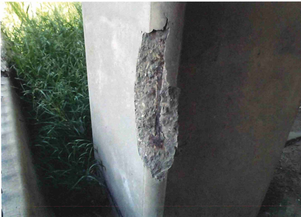
Column (typical) - Typical minor spalling on some of the pier columns.
