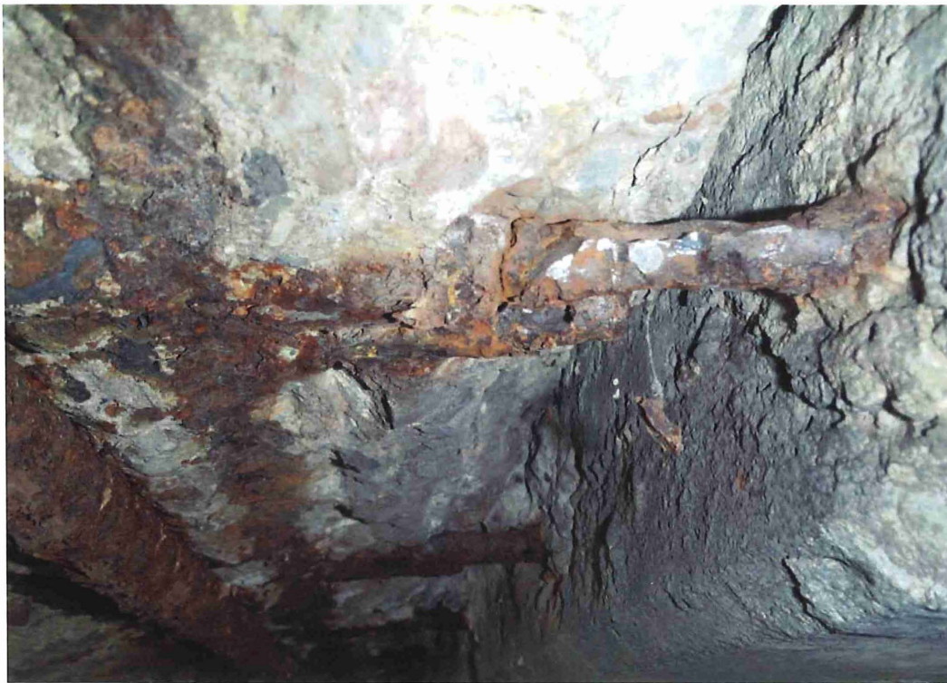
Span 3 - Close up of Broken / 100% section loss in transverse bars.
