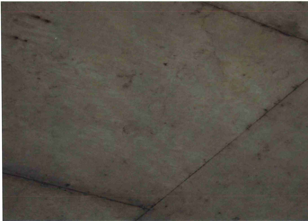
Span 4 - Additional photo of areas of map cracking.
