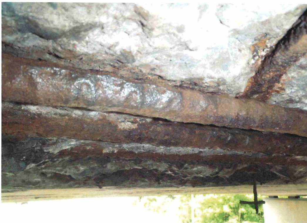
Span 4 - Section loss at midspan of the first rebar, East side of the street.
