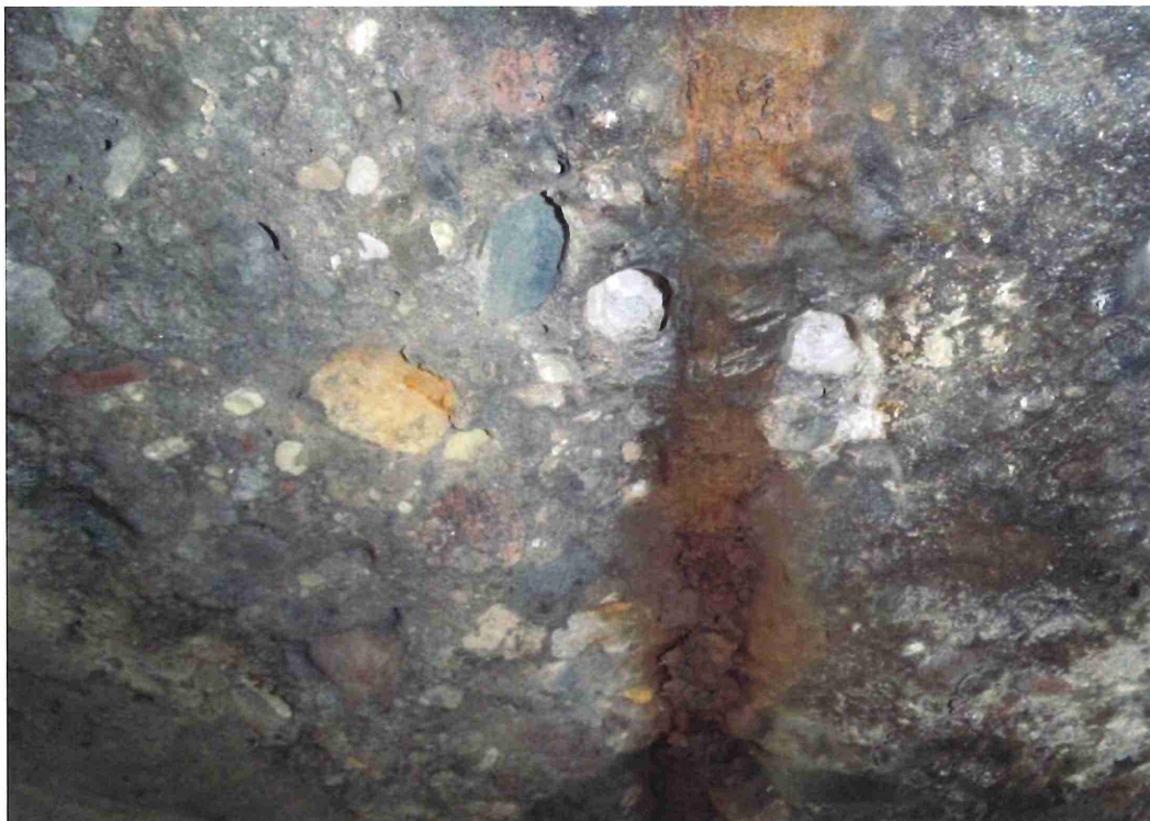
Span 3 - Additional close up of spalled areas occurring in half of span 3
