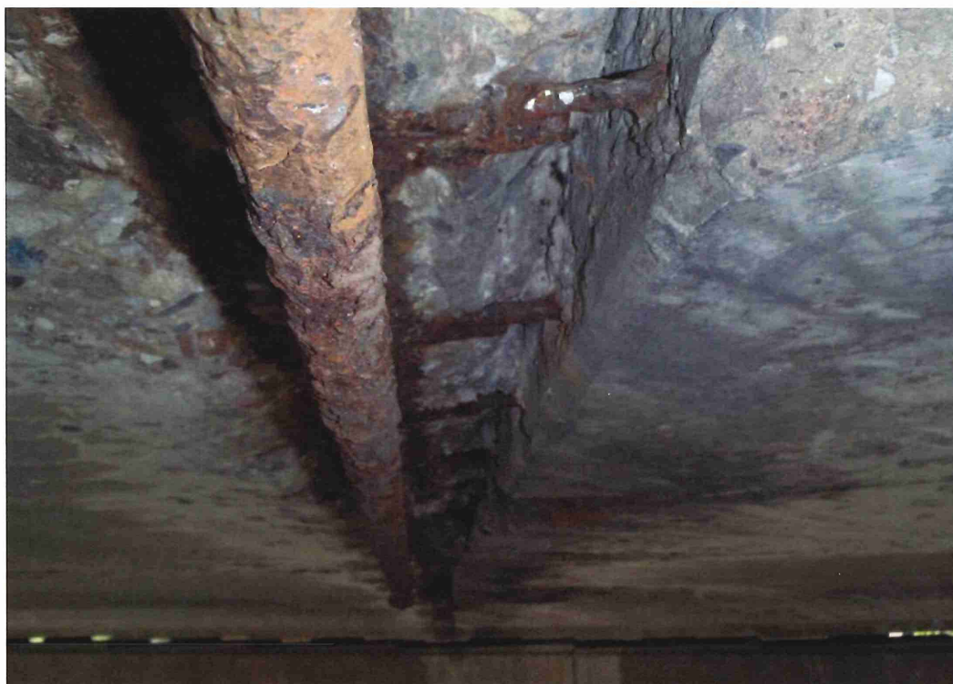
Span 3 - Broken / 100% Section loss in transverse bars.
