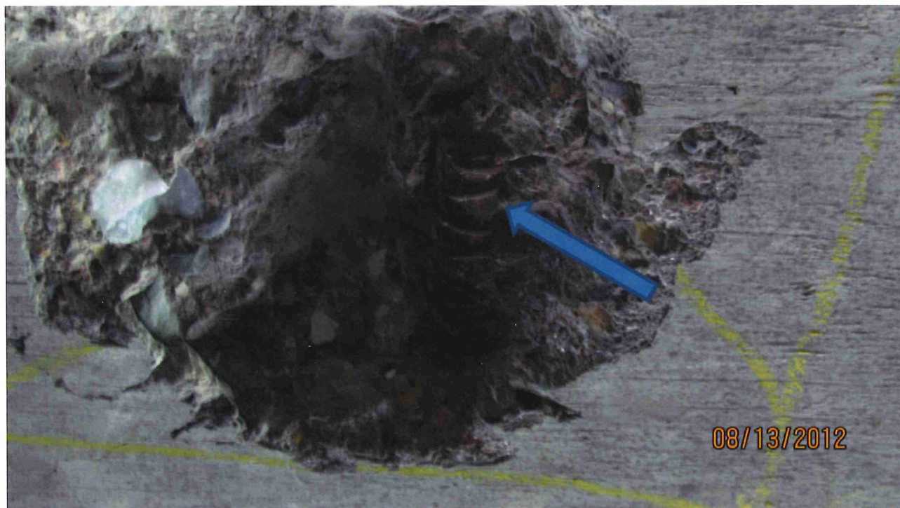
Sample #2 after removal of concrete. There is a light brown staining to the rebar no pack rust or scaling.
