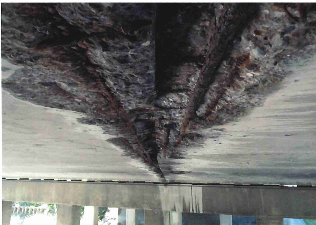
Span 3 - Close-up view of spalled areas. Approximately 2' to 3' either side of centerline joint is either spalled or delaminated full length of span. The exposed reinforcement bars have advanced corrosion with some initial section loss and the spall depth extends up to 3" to 4" deep.
