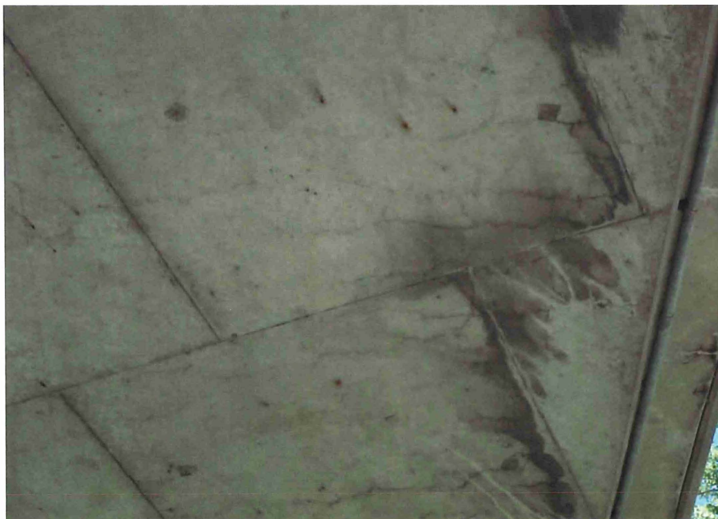
Deck underside (typical) - Additional photo of map cracking along west edge of deck with signs of chloride contamination and staining.
