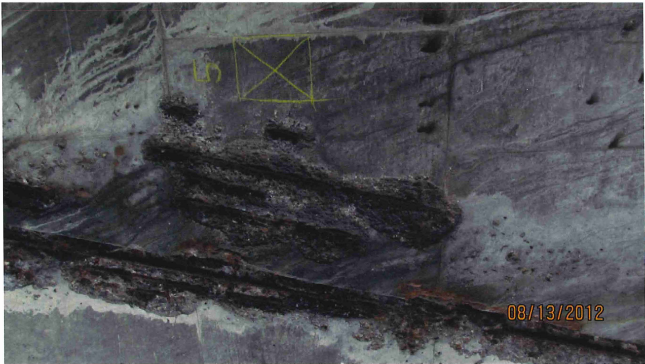
Sample # 5 is 10' North of Pier #2 and 3' west of center line near an area of delamination and spalls.
