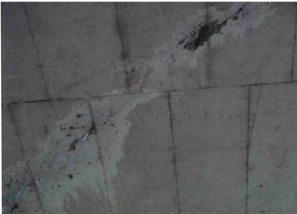
Span 4 - Additional photo of structural crack
