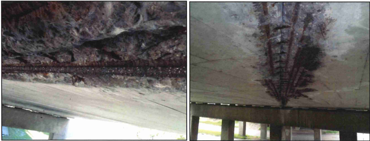
Figure 8. Exposed and debonded reinforcing in Span 3.
