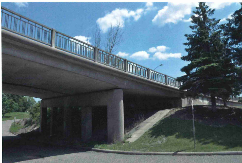
Photo 4. Pier 1, slope paving, and south abutment (facing southeast)
