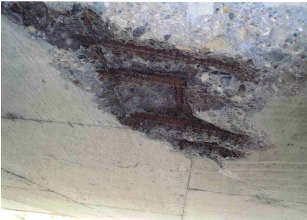
Span 2 - Spalled concrete near Pier 1.
