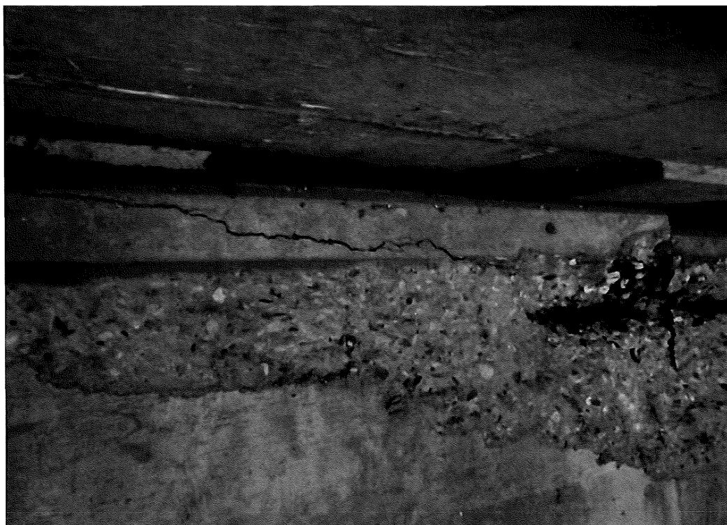
North Abutment - Corner spall/delamination starting at Bearing #3 (from west) and extending to Bearing #5. Spall measures up to 4" deep on abutment face x 16" vertical by 12' long, and delamination on top of cap in same location extends to 8" deep.
