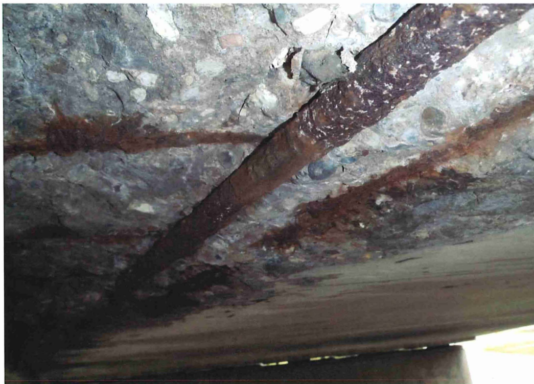
Span 3 - Section loss in two bars, 7/8" remain, starts 12' from Pier 3 and continues to midspan.
