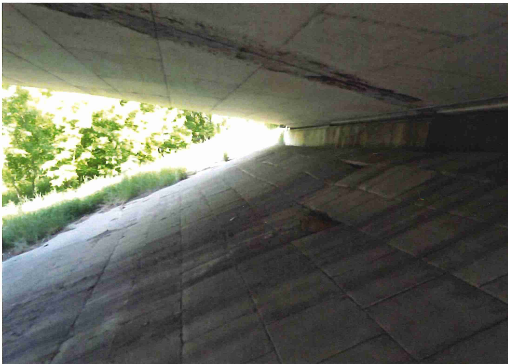
North Abutment slope paving - Slope paving has several areas of severe settlement up to 12".
