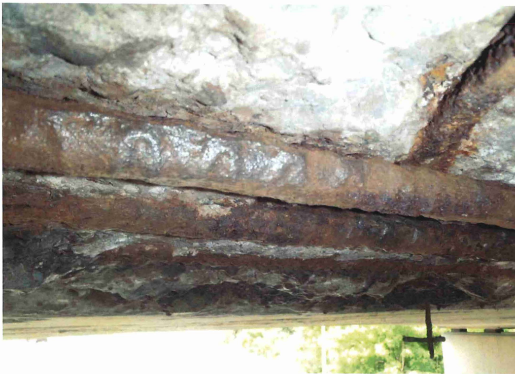
Span 4 - Close up of section loss at midspan, West side of the street.
