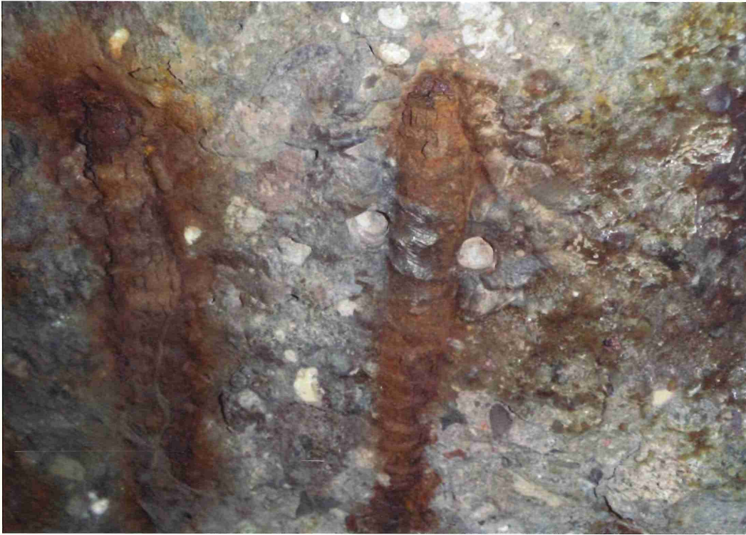
Span 2 - Close up view of spalling in areas of Span 2.
