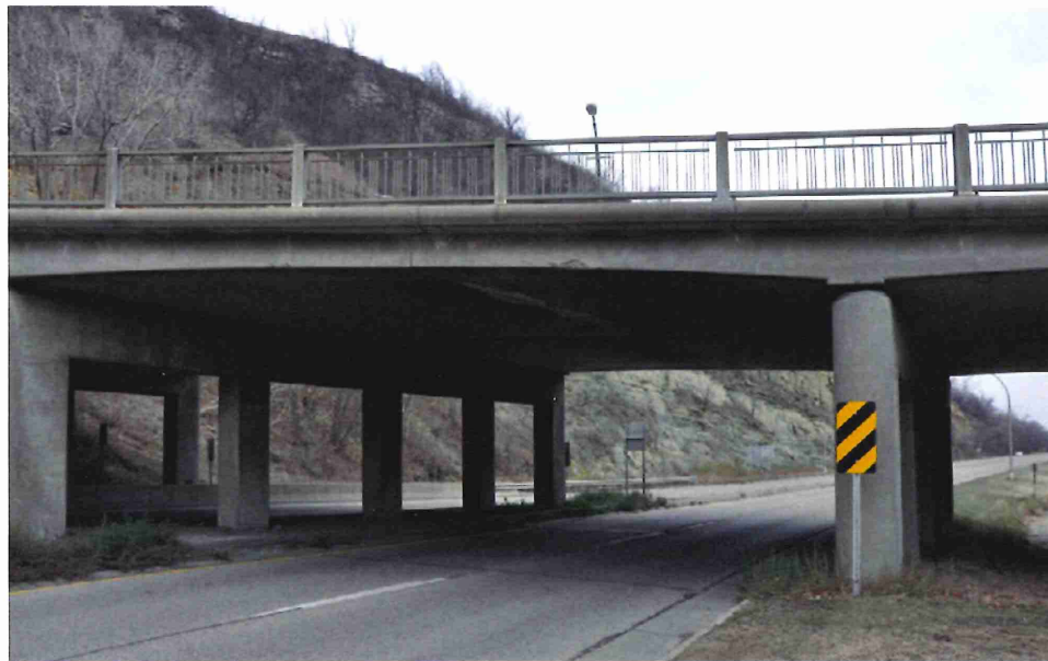
Photo 6. Span 3 and TH 61 southbound lanes; note vehicle damage on slab fascia (facing east)
