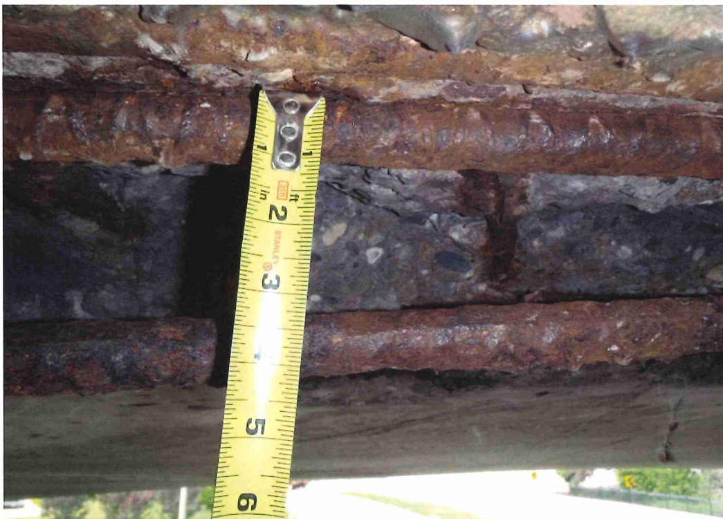
Span 3 - Section loss in two bars, 7/8" remain. Loss starts 12' from Pier 3 and continues to midspan
