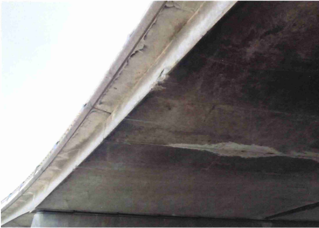
West fascia - Minor impact damage on west fascia above the SB 61 lanes.
