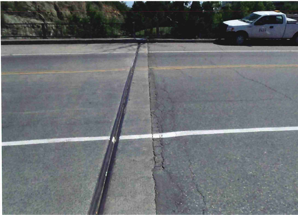
South approach pavement - Minor settlement and poor condition of bituminous pavement noted.
