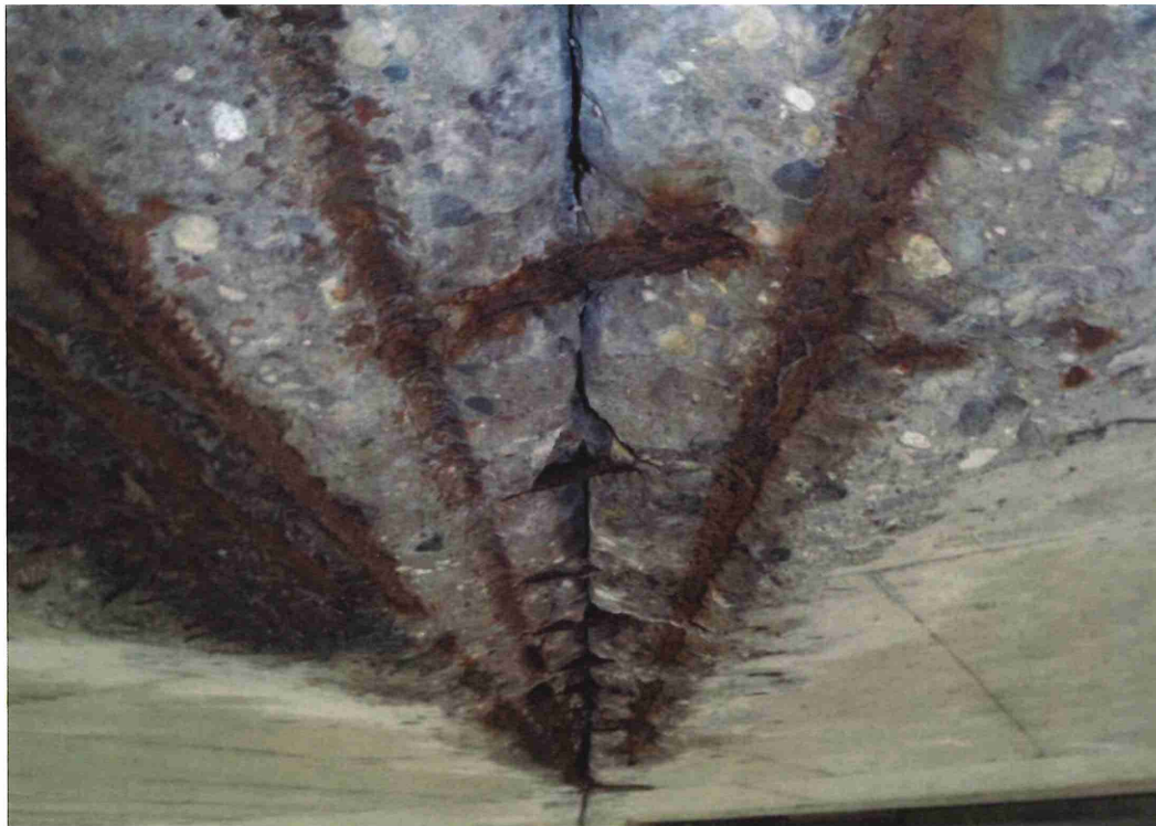
Span 4 - Missing rebar along 2/3 of span.
