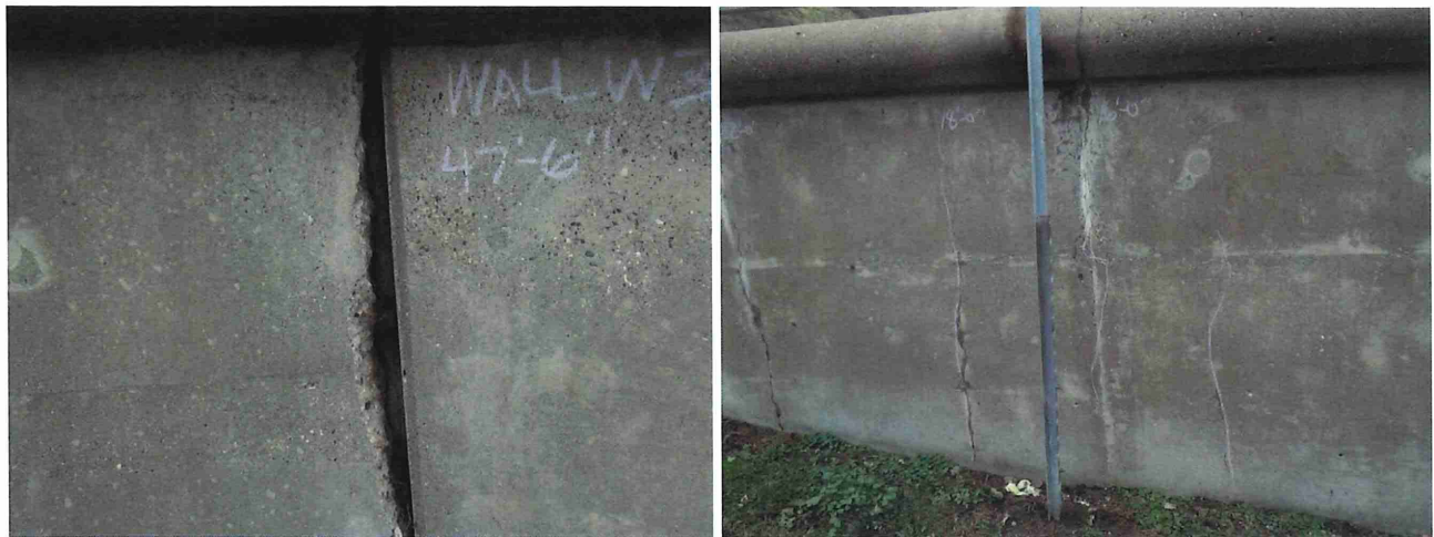
Figure 10. Typical spalls and cracks in the approach retaining walls.
