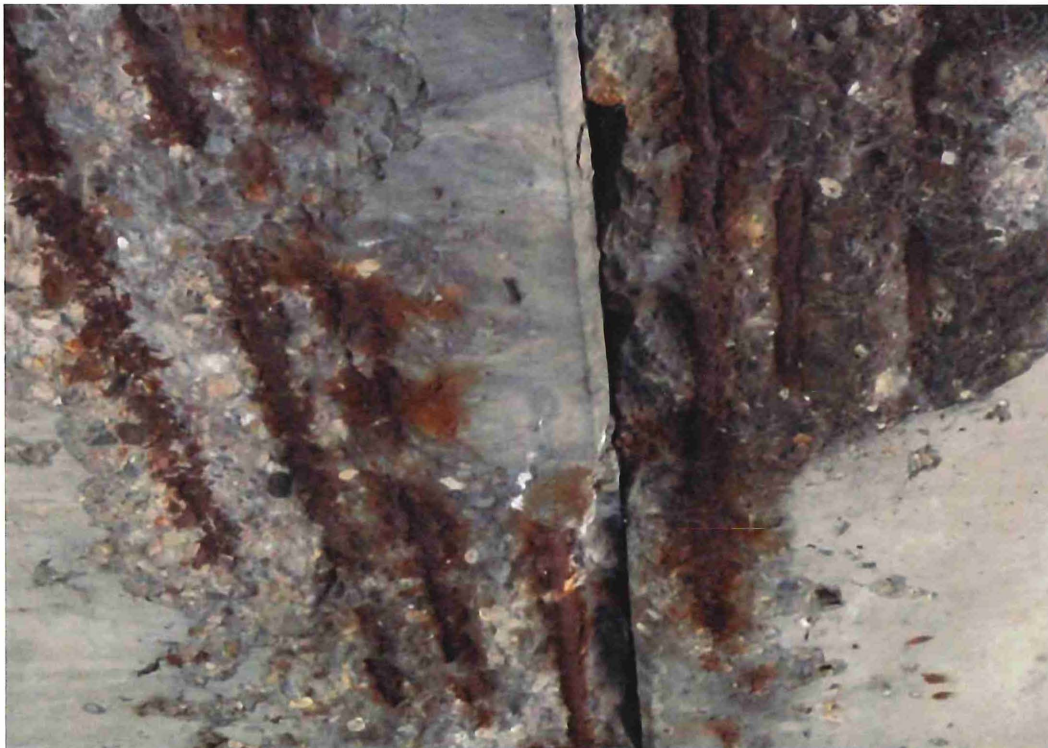
Span 2 - Additional close-up view of spalled areas.
