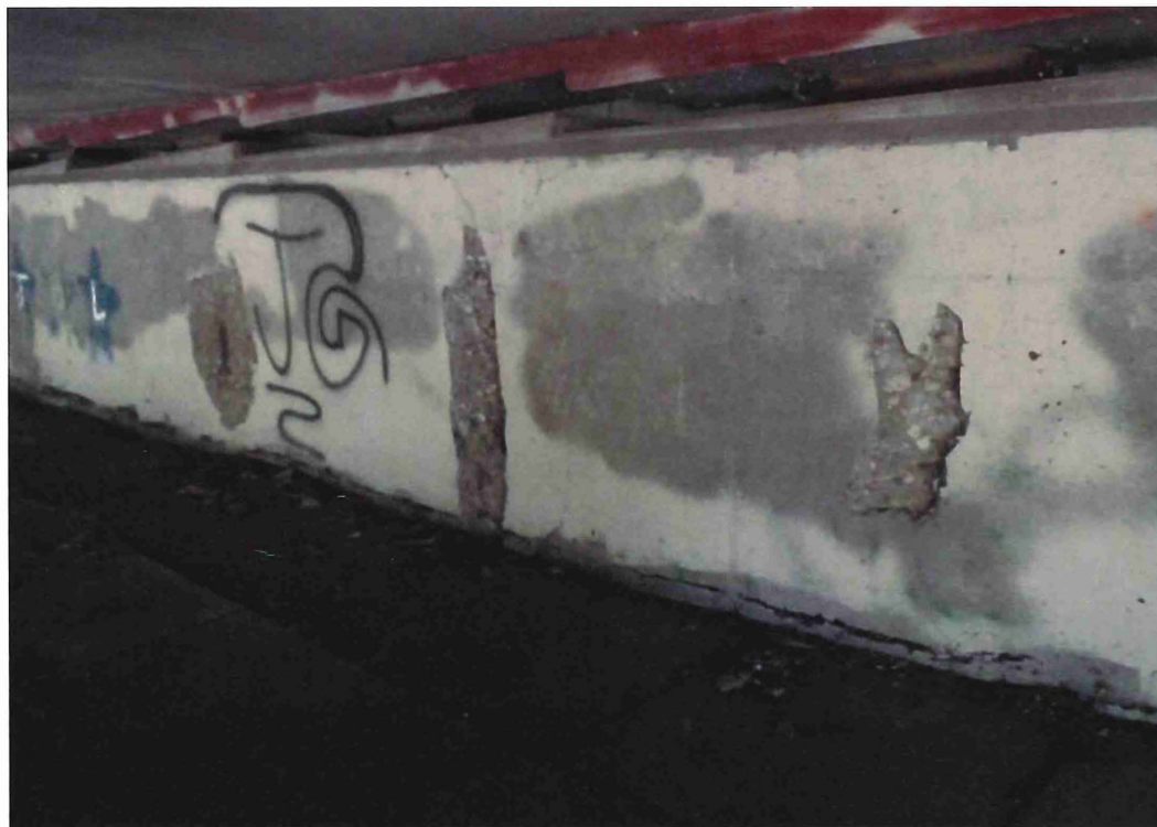
South Abutment - Several areas of spalling extending to 2" deep with some exposed reinforcement bars.
