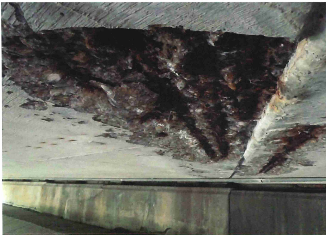
Span 5 - Close-up view of spalled areas. Approximately 2' either side of centerline joint is either spalled or delaminated full length of span. The exposed reinforcement bars have corrosion with some initial section loss and the spall depth extends up to 3" deep.
