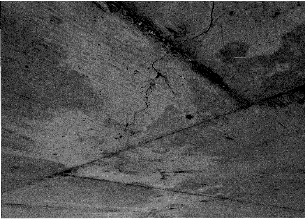
Span 4 - Close up view of hairline crack.
