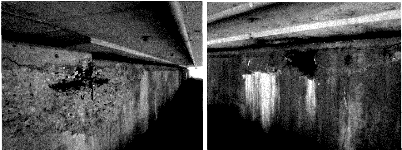
Figure 9. Spalled and delaminated concrete on the north abutment.
