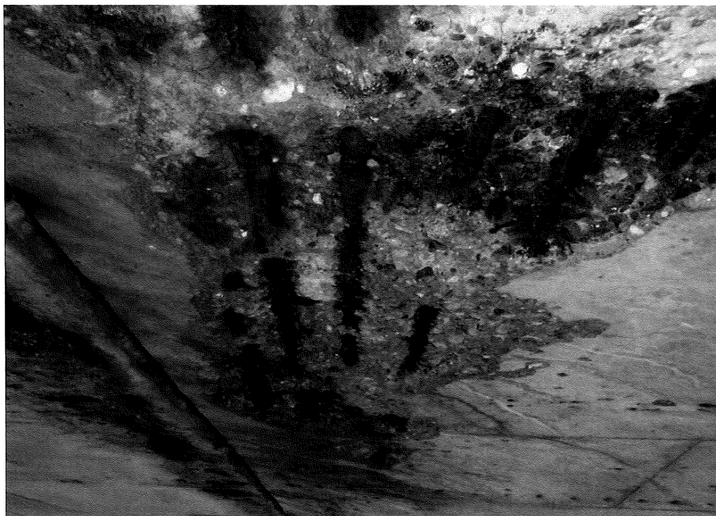
Span 2 - Section loss and spalling in areas of Span 2.
