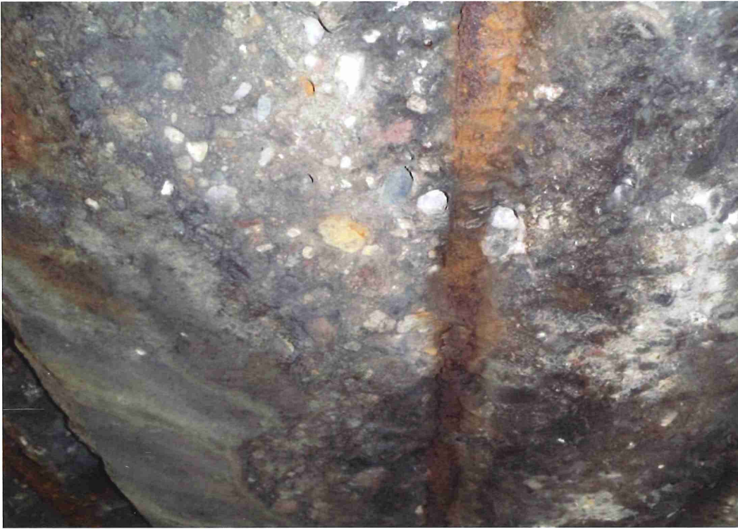
Span 3 - Close up of spalled areas occurring in half of span 3
