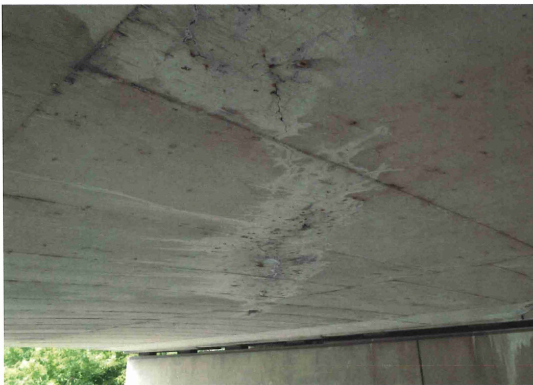
Span 4 - Hairline crack with efflorescence. The concrete is sound around the crack.
