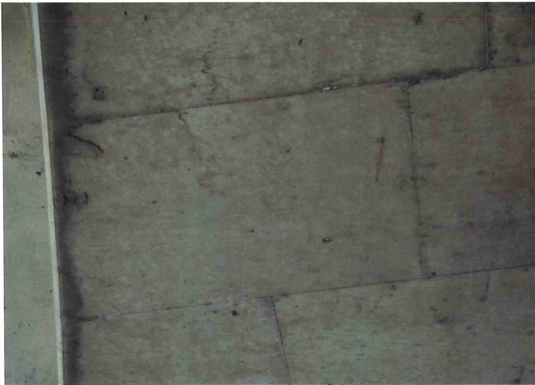
Deck underside (typical) - Map cracking along west edge of deck extending in approximately 4'-0" with signs of chloride contamination and staining.
