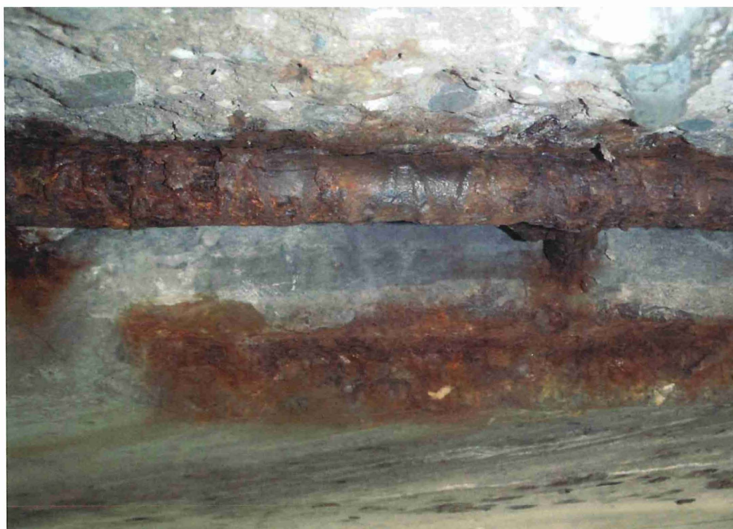
Span 3 - Section loss at the South end of the span.
