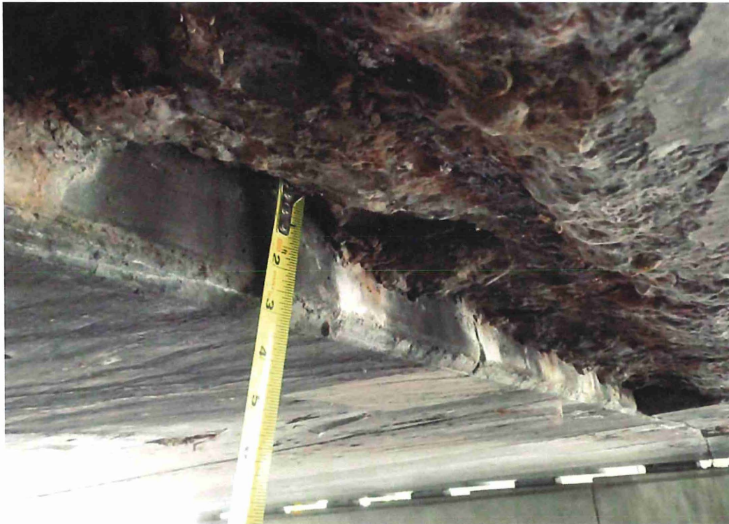
Span 1 - Close-up view of spalled areas. Approximately 2' either side of centerline joint is either spalled or delaminated full length of span. The exposed reinforcement bars have corrosion with some initial section loss and the spall depth extends up to 3" deep.
