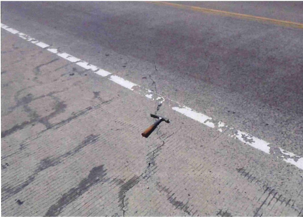
Deck surface, Span 5, NB lane - Structural crack with delamination along length.
