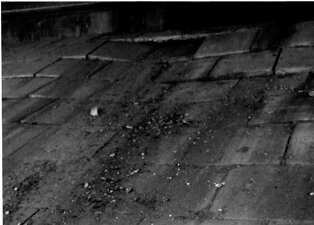
North Abutment slope paving - Additional photo of severe settlement.
