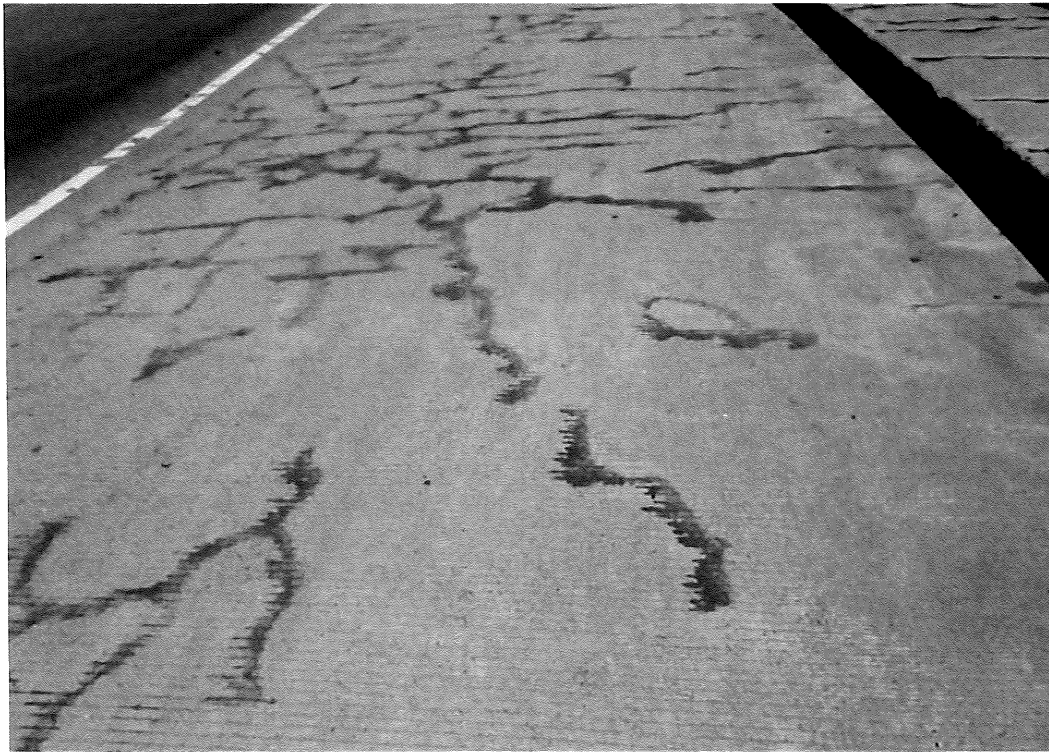
Deck surface - Map cracking on deck surface (NB lane shown, typical throughout).
