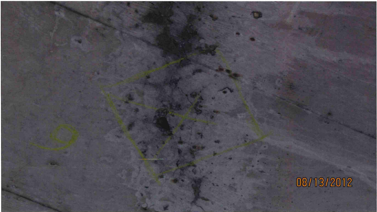
Sample # 6 is 16' 5" South of Pier #4 and West 5' of center line. This location show signs of cracking and pour consolidation of concrete.
