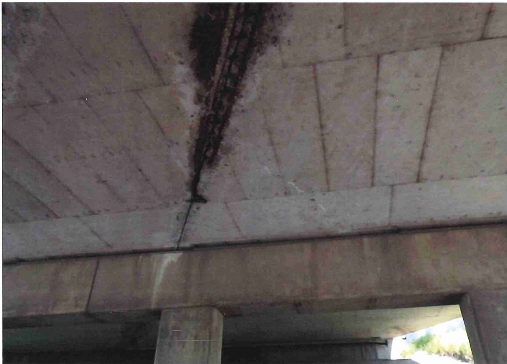
Span 4 - Diagonal structural crack with efflorescence starting 24' from the east edge of deck at Pier 4, and extending to the CL bridge joint 12' from Pier 4.
