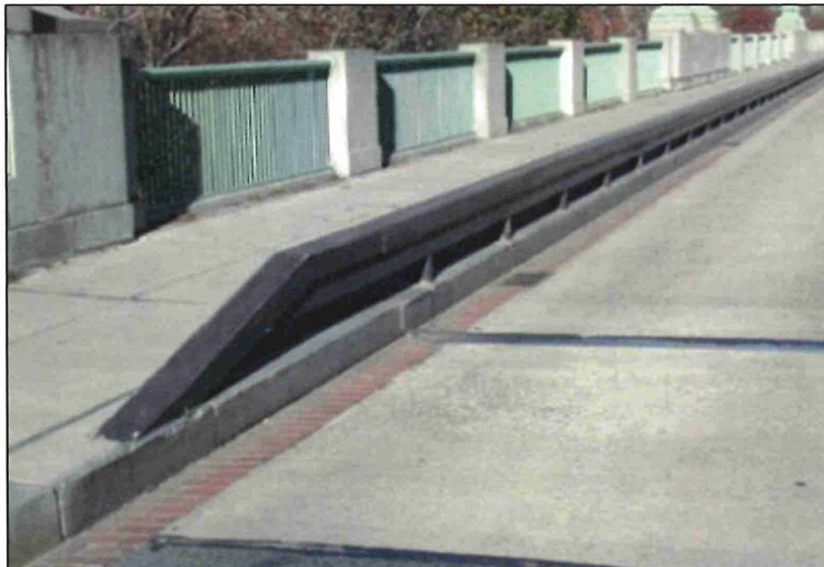
Figure 14. Inner TL-2 rail used in Washington, DC. This information, included in FHWA's 2005 Bridge Rail Guide, shows the rail mounted on the Taft Bridge on Connecticut Avenue in Washington, which is listed on the National Register.
