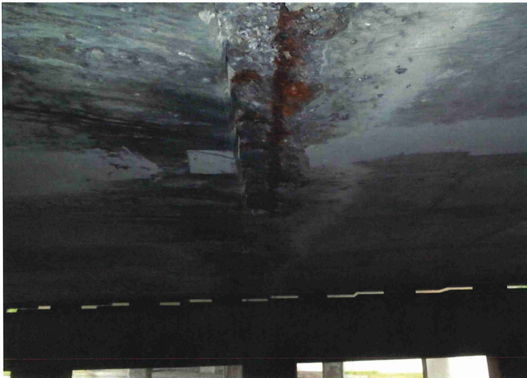
Span 1 - Spalling in the interior of Span 1.
