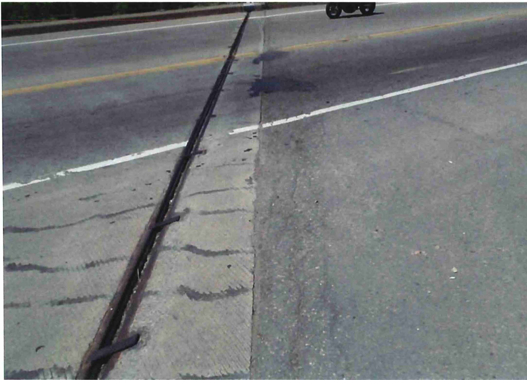
North approach pavement - Evidence of settlement full width of approach.
