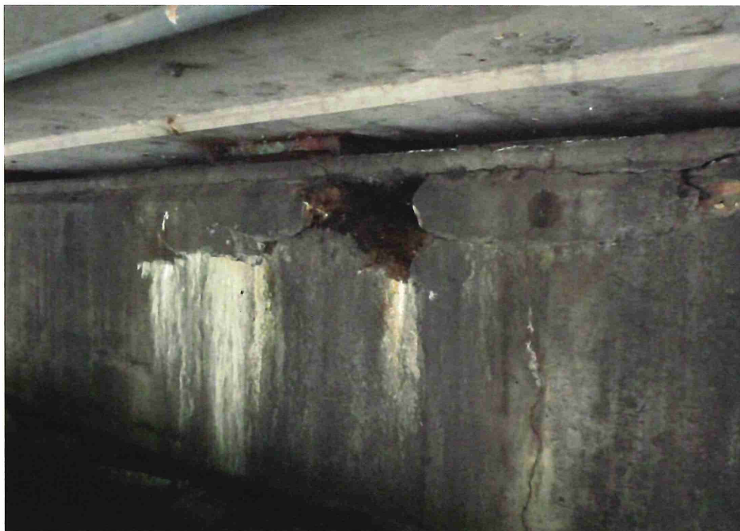
North Abutment - Corner spall/delamination between Bearing #8 (from west) and Bearing #9. Spall measures up to 3" deep on abutment face x 12" vertical by 6' long, and delamination on top of cap in same location extends to 4" deep.
