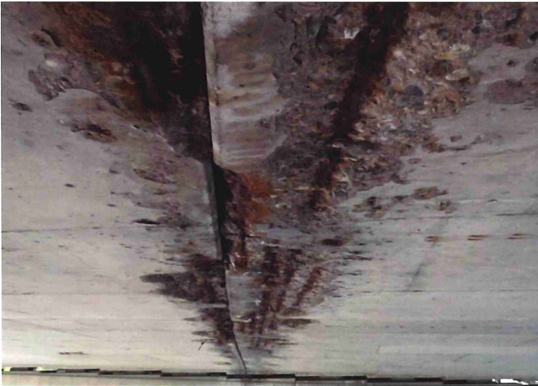
Span 2 - Close-up view of spalled areas. Approximately 2'-6" either side of centerline joint is either spalled or delaminated full length of span. The exposed bars have corrosion with some initial section loss and the spall depth extends up to 3" deep. Some loss of bond is occurring on some longitudinal reinforcement bars.
