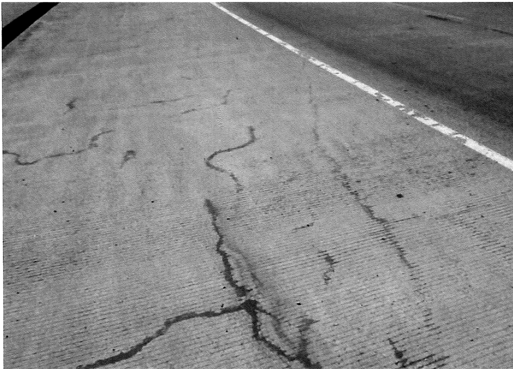
Deck surface, Span 2, NB lane - Structural crack with delamination along length.
