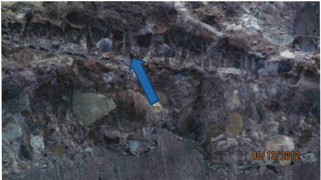
Sample # 5 after removal of concrete. Rebar shows no sign of rust.
