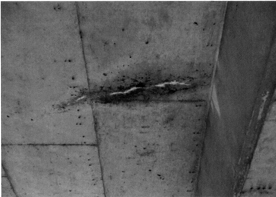
Span 4 - Close up view of hairline crack.
