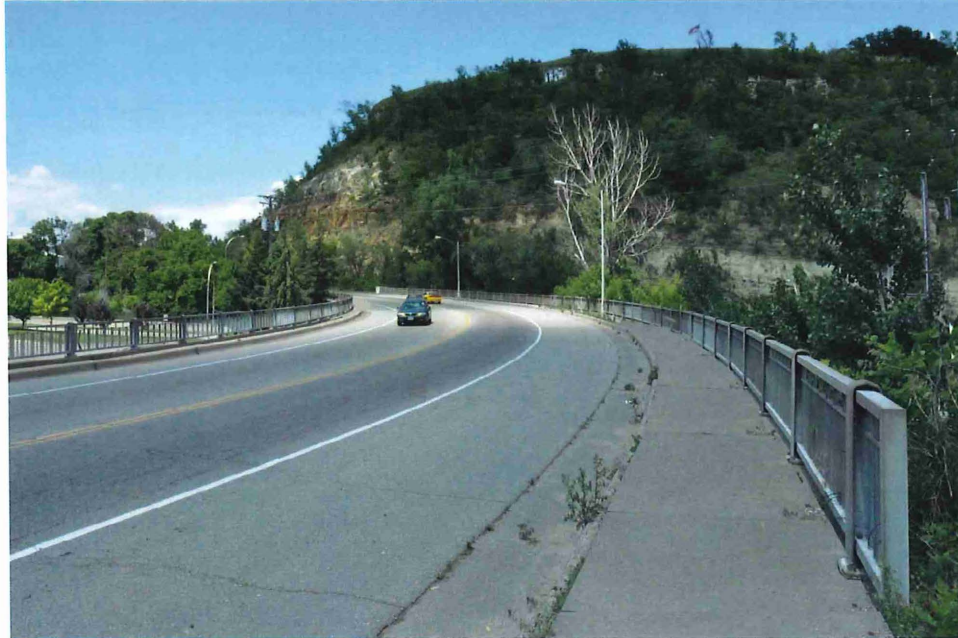
Figure 16. Bridge 9103 “before” the addition of the proposed inner TL-2 railing.
