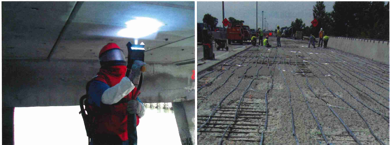
Figure 13. Cathodic protection: arc-spraying a zinc coating (left) and embedding sacrificial anodes in the top of a slab (right).
