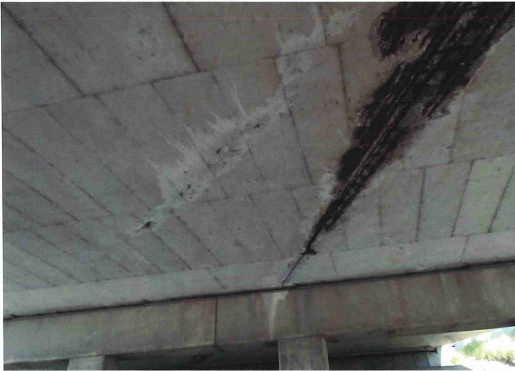
Span 4 - Circular structural crack with efflorescence starting 20' from the west edge of the deck at Pier 4, and extending to the CL bridge joint at approximately the midspan of Span 3.
