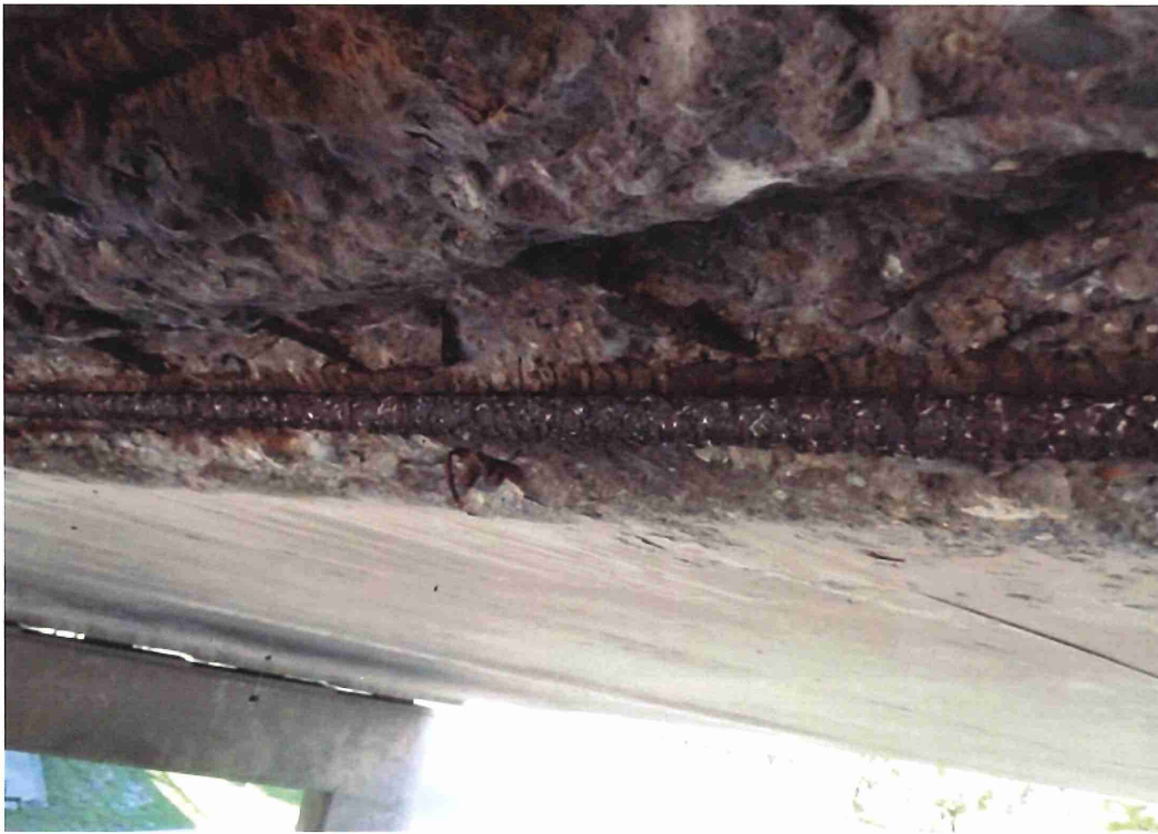
Span 3 - Close-up view of spalled areas. Some loss of bond is occurring on four longitudinal reinforcement bars. One longitudinal bar with 3/4" remaining section.
