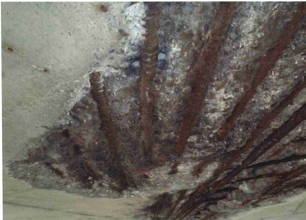
Span 4 - Spalled deck area with 6 exposed rebar measuring 1" in diameter.
