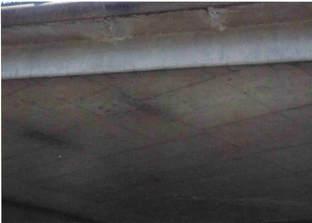
West fascia (typical) - Vertical hairline cracks at approximate 12" centers (typical).
