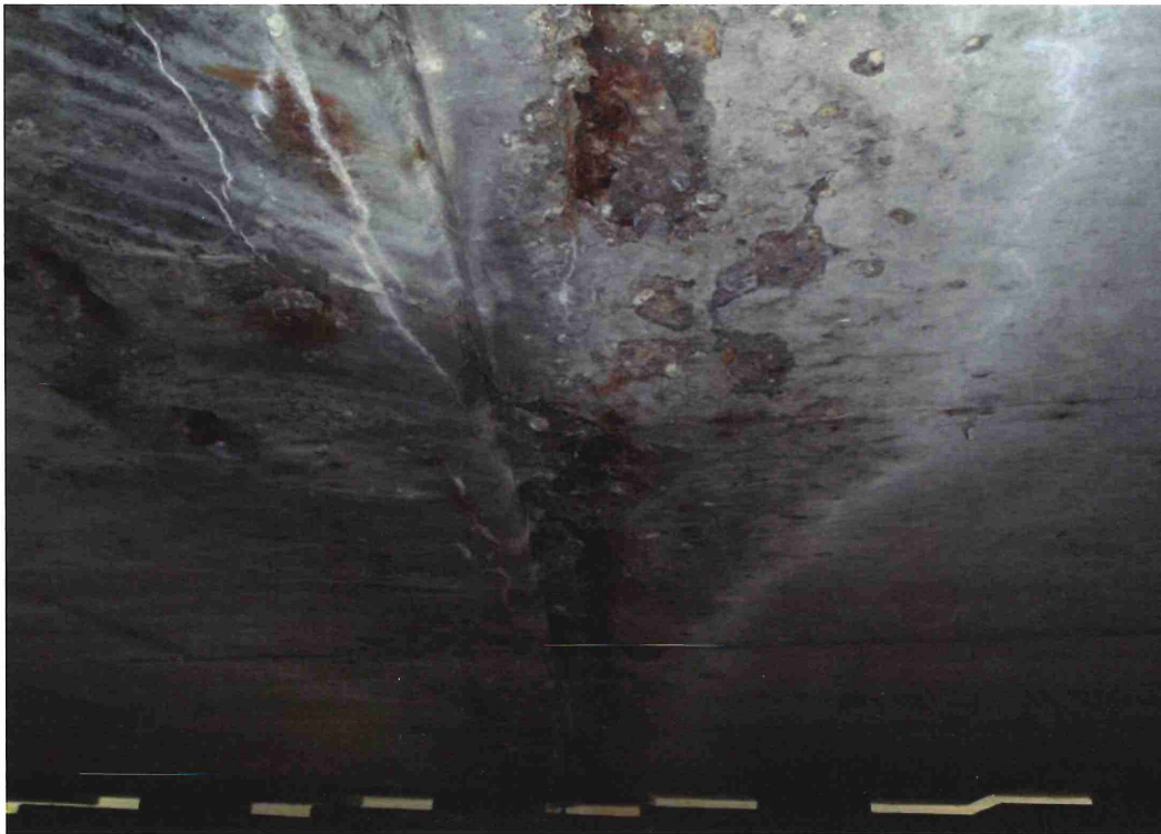
Span 1 - Additional photo of spalling in the interior of Span 1.
