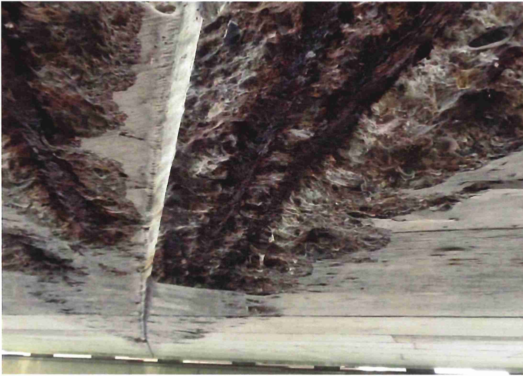
Span 5 - Additional photo of spalled areas.
