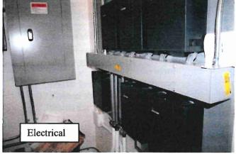
enclosure and has spare breakers for future expansion. Barracks building has a Siemens fire alarm panel. Facility is in the process of completing installation of a new IP camera and recording system. System is expandable to accommodate additional cameras in the added and remodeled spaces. All equipment is from the original construction and has been well maintained and is in good condition.
