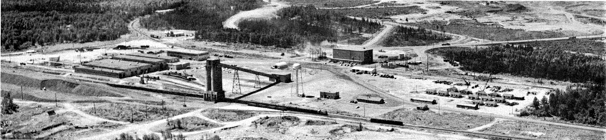
RESERVE MINING COMPANY'S TACONITE QUARRY AND PRIMARY CRUSHING PLANT AT BABBIT — Upper right shows quarry where crude taconite is mined and is then hauled to primary crusher shown in center and what appears to be two silos to the left are storage bins where the ore is received from the crusher and loaded into the railroad cars to be hauled 47 miles to Silver Bay. Under Reserve's 120 million dollar expansion program, these units will be duplicated at Babbitt; the railroad will be double-tracked and the processing units at Silver Bay will also be expanded to increase the present capacity by 50 per cent to 9 million tons of pellets per year.
