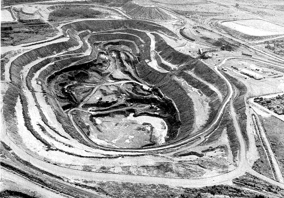
STATE-OWNED OPEN PIT MINE AT HIBBING — Operated by Morton Ore Company (The M. A. Hanna Company, Agents). Haulage incline, concentrating plant, shops and tailings pond to the right, and waste material stockpiles in the background.
