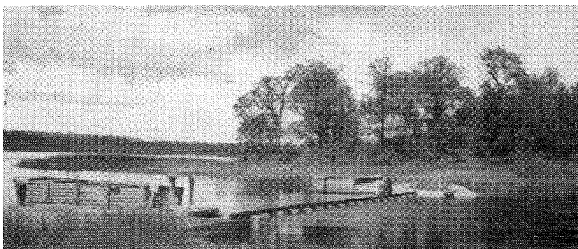
Dam with Carp-Control Device on Ogechie Lake. This dam controls the water level of Mille Lacs Lake; also stops migration of carp into Mille Lacs Lake.
