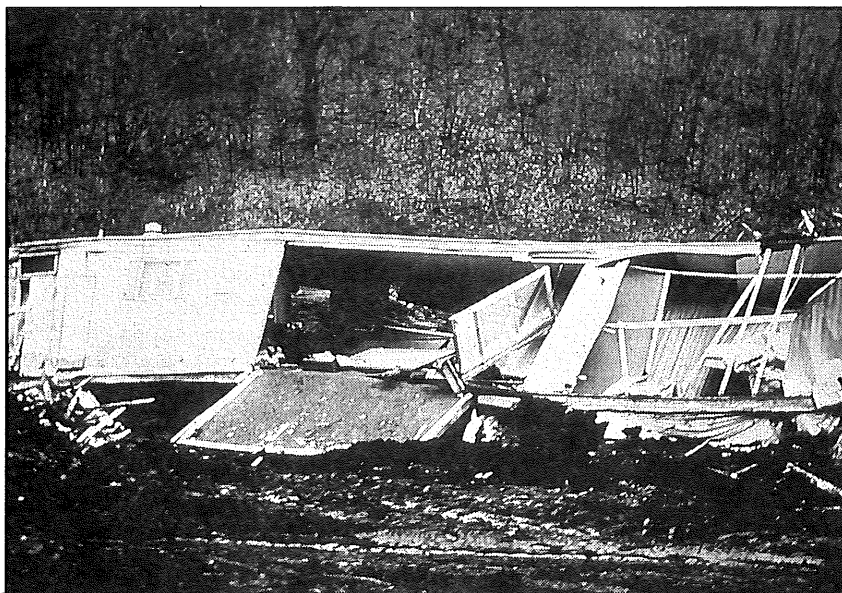
Figure 6.2 By adhering to floodplain guidelines for the placement of manufactured homes, owners can avoid expensive flood damage.
