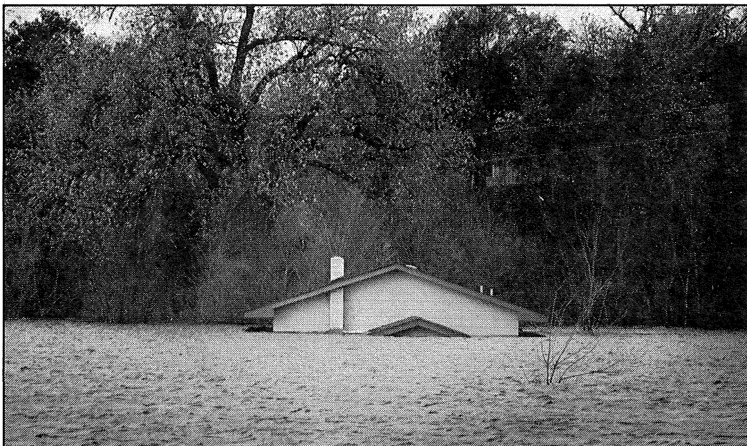
Figure 7.2 Proper ordinance administration can save lives and prevent property damage.
