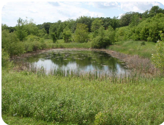
Figure 4. Stormwater retention pond in Scott County.
