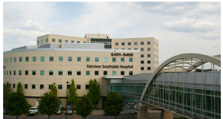
Figure 9. Fairview Southdale Hospital in Edina, MN
