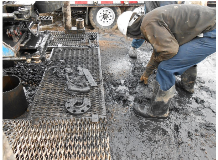
Removing debris from the Marshall Processing Plant well in preparation for sealing.
