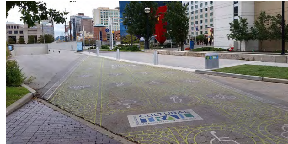
Textured pavement demarcates the conflict zones between automobiles and trail users.
