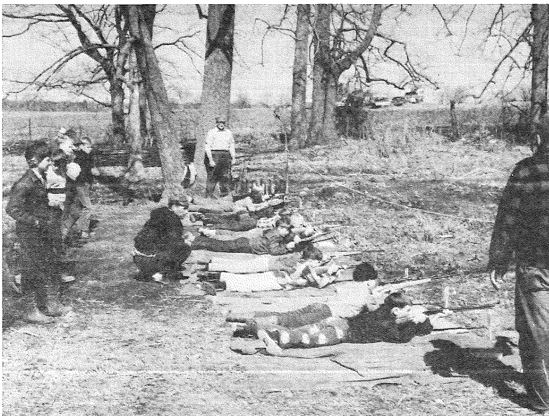
More than 51,000 youths were trained in the safe handling of firearms under the Youth Firearms Safety Training Program of the Division of Enforcement and Field Service.
