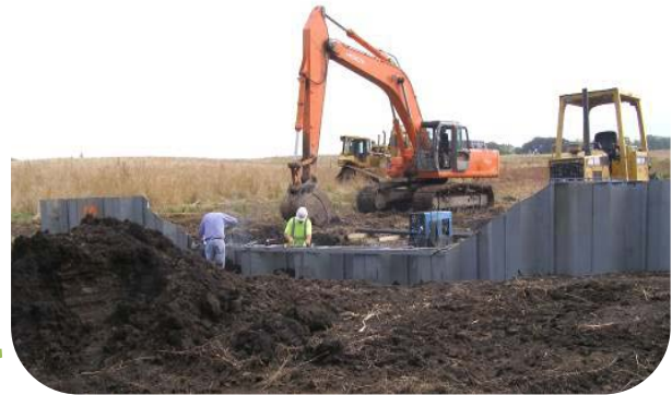
Cutting and shaping top for cap installation.
