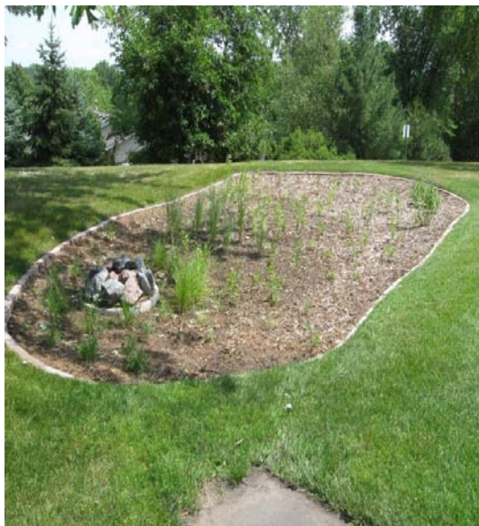
Hoffman raingarden in Shoreview, constructed in 2008. Project funded by cost-share funding from the Grass Lake WMO and RCD. The raingarden manages urban runoff from 2/3 acre.
