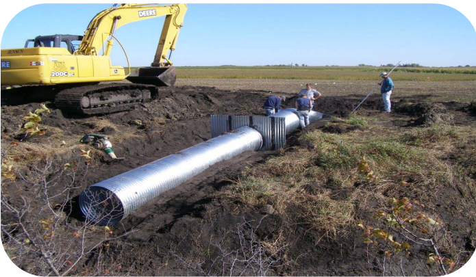
Pipe assembled and ready for backfilling.
