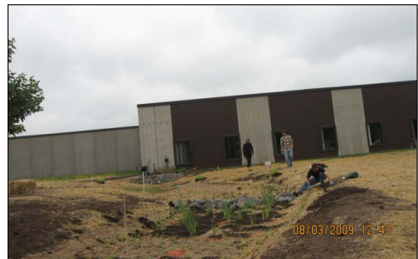
Miller Creek Restoration Irresistible Ink stormwater control bio-retention swale
