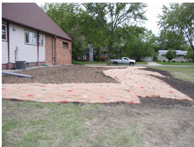
Rain Garden Installed at Christ Lutheran Church in Glencoe.
