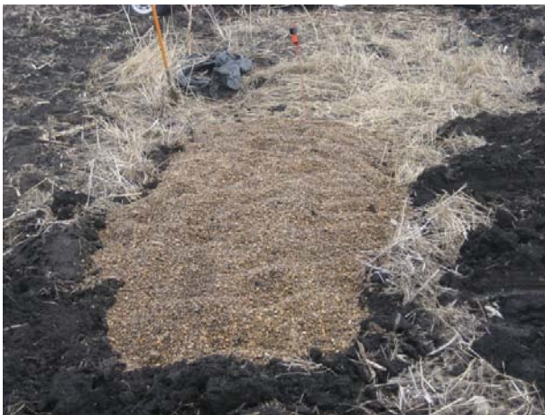
Pictured: Rock tile inlet installed by a local landowner. Inlet was later planted with a 10 foot grass buffer.
