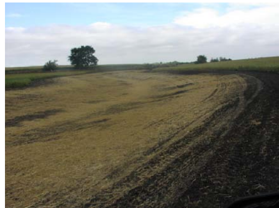
Waterway ~ seeded and mulched, the picture above was taken right after construction
