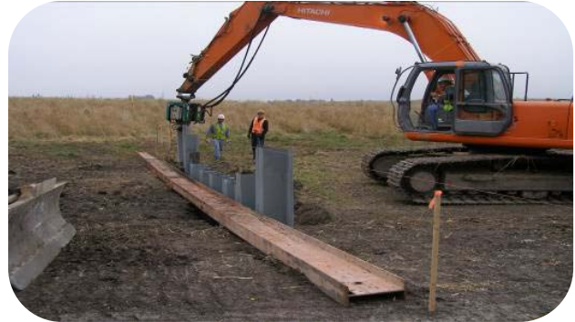
Driving steel sections of a Sheet Pile Structure. Backhoe on right, Steel I beam on ground, string for
