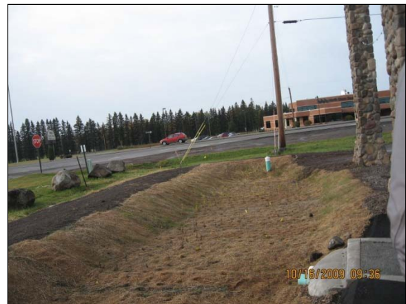
Miller Creek Restoration Energy Plus stormwater control bio-retention basin
