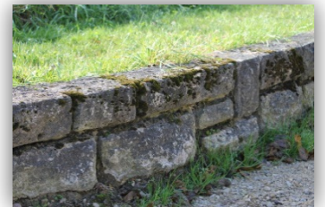
Stone curb at Meadow Trail parking lot
