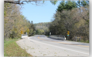
TH 74 bridge over the Whitewater River
