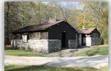
Combination building exterior
