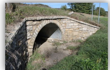
WPA-constructed culvert in the new campground area
