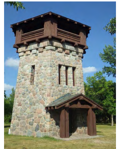
The combination water and observatory tower is a contributing structure to the historic district.
