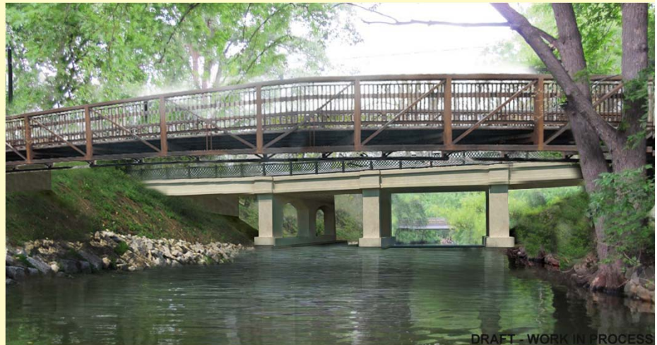
Pedestrian and bicycle bridge Vaulted steel structure, no in-channel piers
