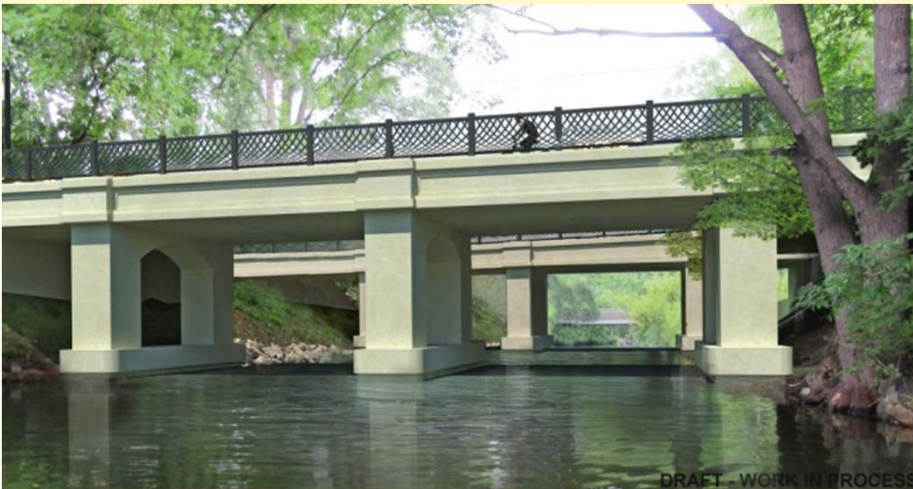
Modified SPO bridge Concrete arched in-channel piers
