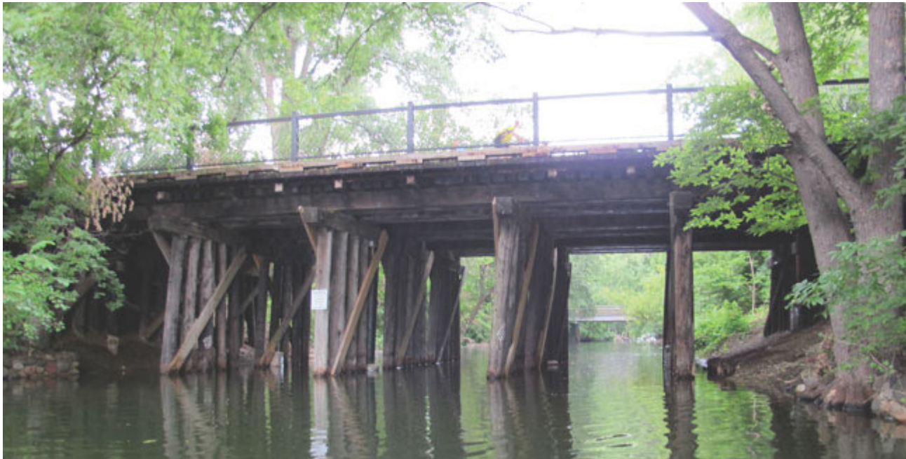
EXHIBIT 5 PHOTO OF THE EXISTING BRIDGE OVER THE CHANNEL
