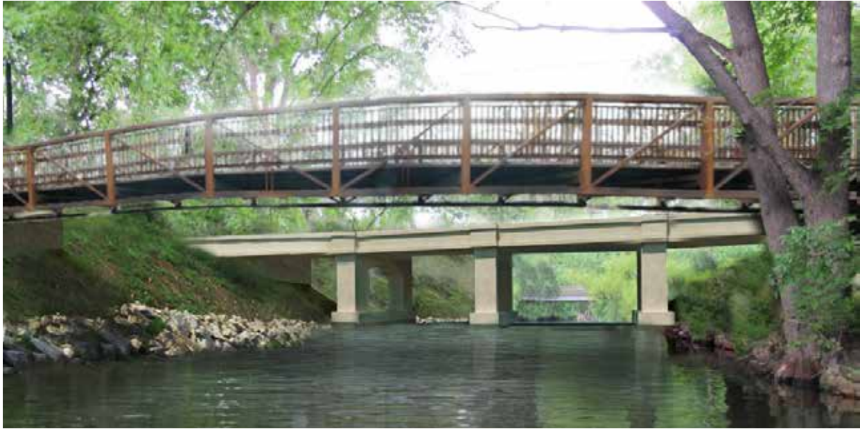
Depiction of a 'lightweight' pedestrian truss bridge used as a visual impact mitigation measure for the Kenilworth Channel crossing.
