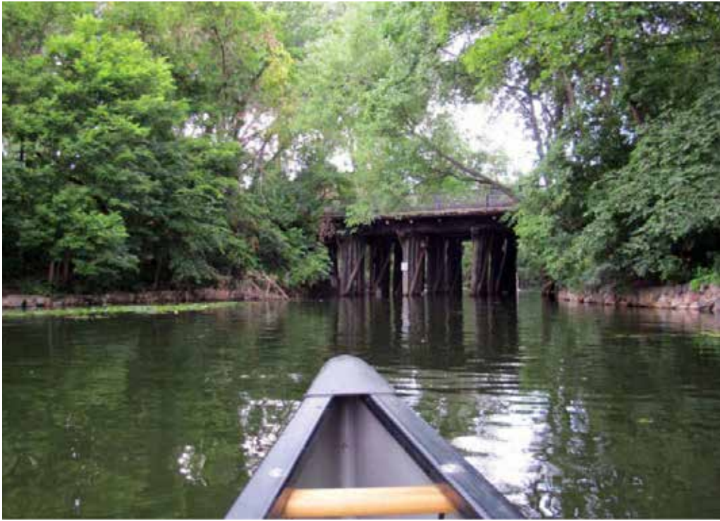
a. Photograph of the existing view looking northwest from the Kenilworth Channel/ Lagoon toward the freight rail and trail trestle bridges.
