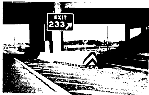
Impact attenuators and other safety improvements can affect the appearance of existing highways to which they are added.
