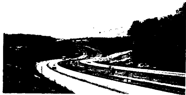
Horizontal and vertical curves have been coordinated on this freeway, making it appear to flow smoothly over the rolling landscape, despite the high design speed.
