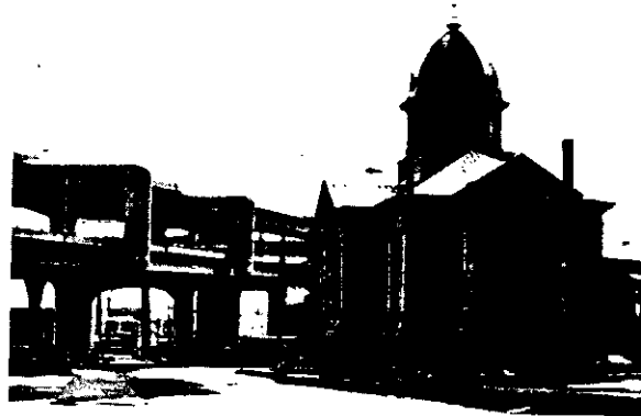
Despite considerable design effort, this bridge approach structure does not succeed in eliminating adverse visual effects on the church next to it.
