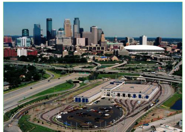
Above: The Franklin Operation and Maintenance Facility, serving the Blue Line (Hiawatha LRT), features on-site parking for staff and fully enclosed storage areas for light rail vehicles.
