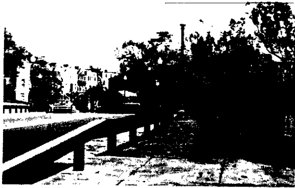
A steel guard rail was carefully designed to complement the visual character of this historic bridge after the appearance of a concrete barrier proved unsatisfactory.
