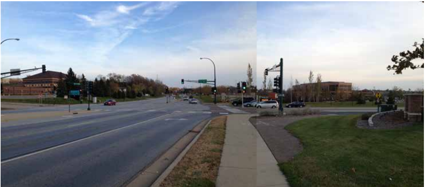
a. Photograph of the existing view looking south along Prairie Center Drive at Technology Drive toward the proposed alignment of elevated LRT structure.
