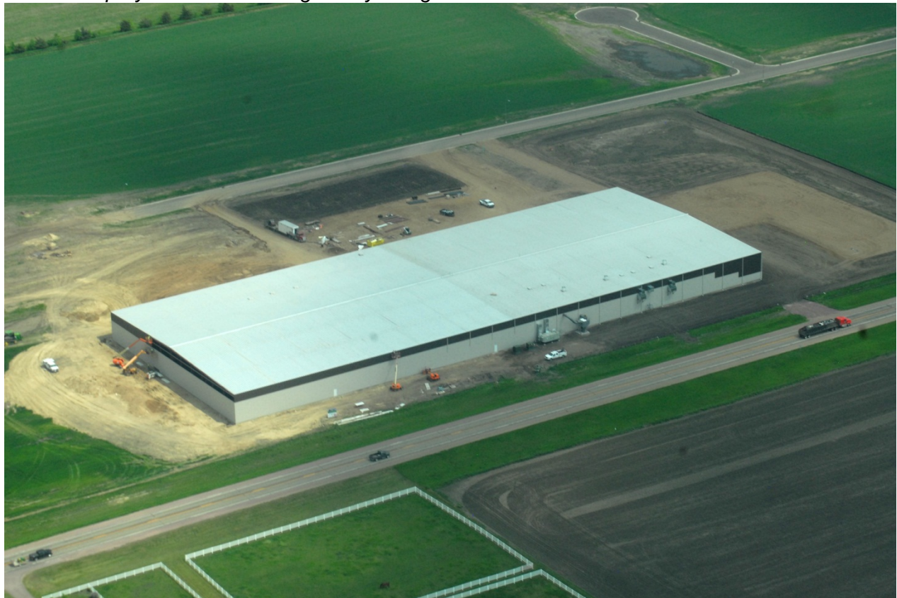
Fast Sprayers manufacturing facility along North Industrial Park access road
