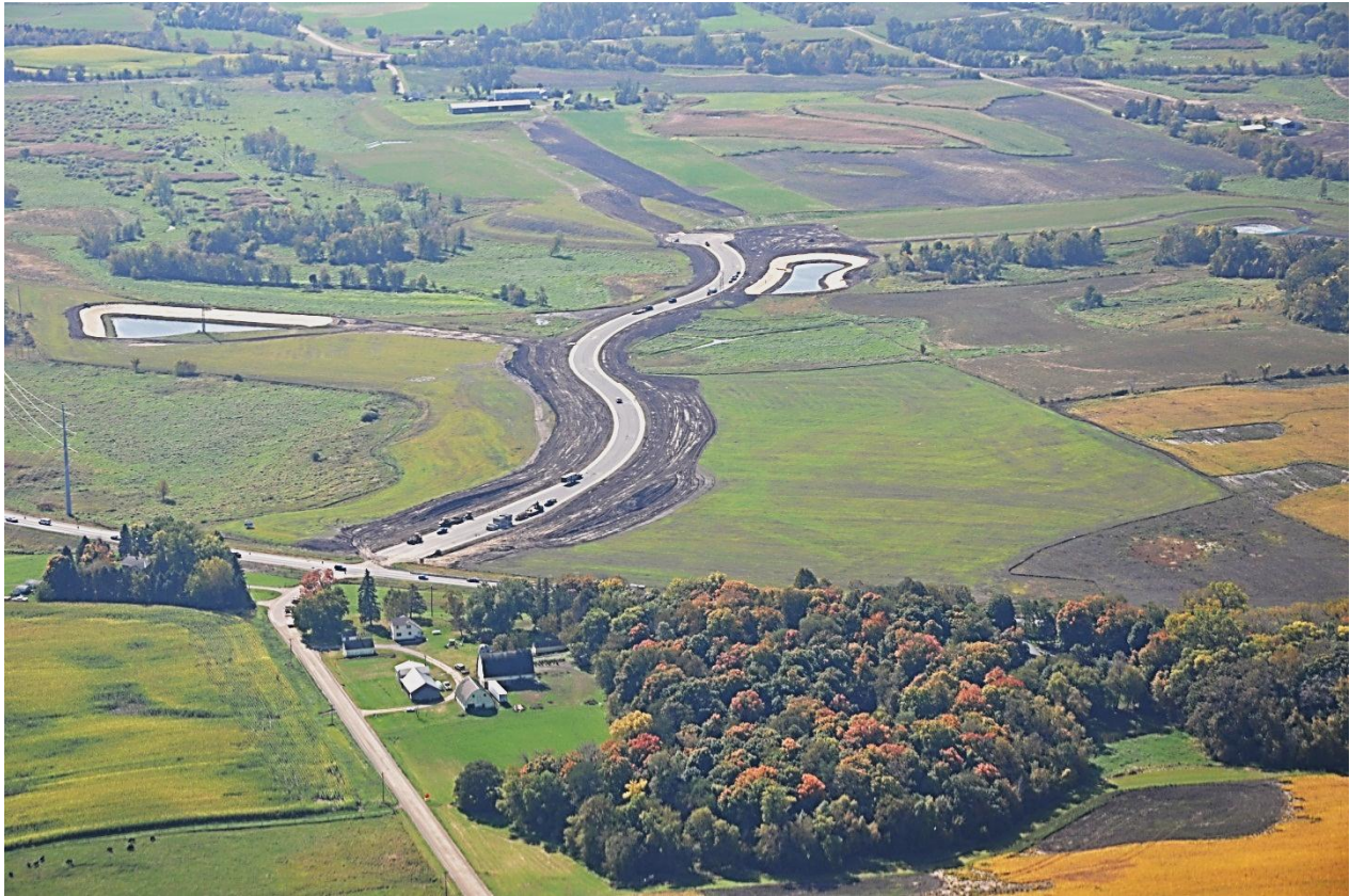
Delano Business Park access road
