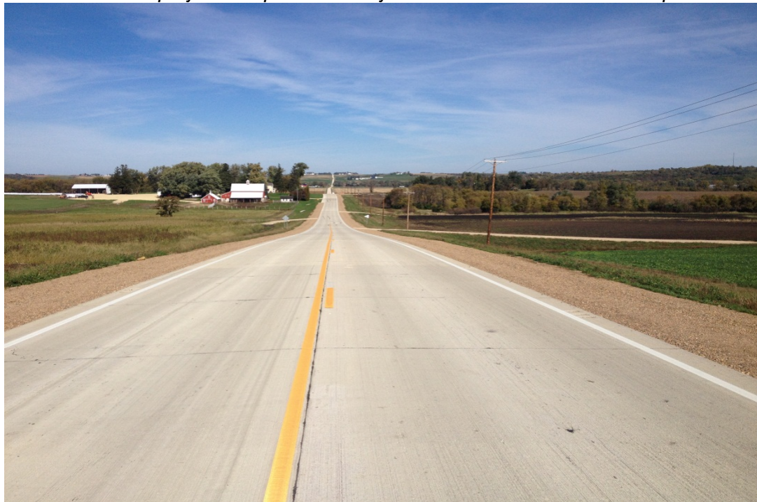
2010 TH 52 project completed in conjunction with the Versa Cold expansion
