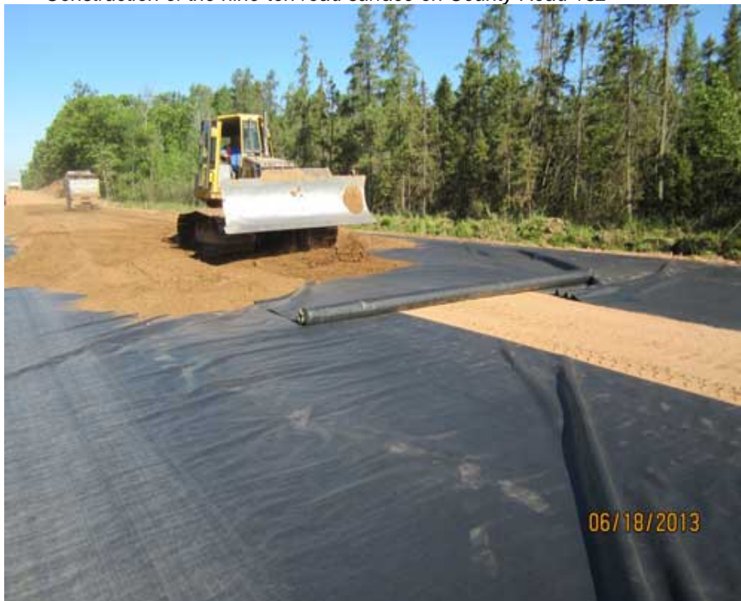
Construction of the nine-ton road surface on County Road 132
