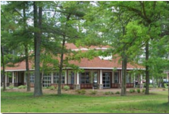
This three-season structure is an example of how expanding on a common picnic shelter theme can bring in new user groups and expand seasons.
