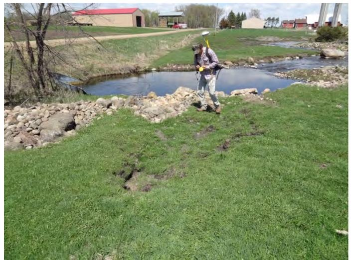
The longest hydrologically connected SPI signature of the top 1% of values in the study area was along Mill Creek (pictured above left). The accompanying field photo shows signs of slumping in the small pasture (foreground) and the landowner had installed rip-rap along the stream bank for stabilization. There was no further evidence of erosion upland of the slumping.
