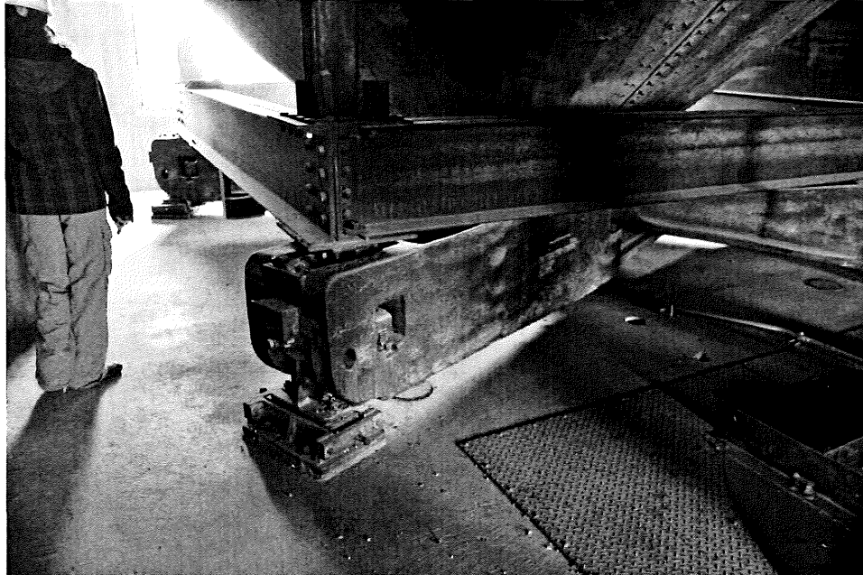
Fig. 208. 810 Levee Rd. Burdick Grain Co. Terminal Elevator, base of the hopper scale on the scale floor (facing S)
