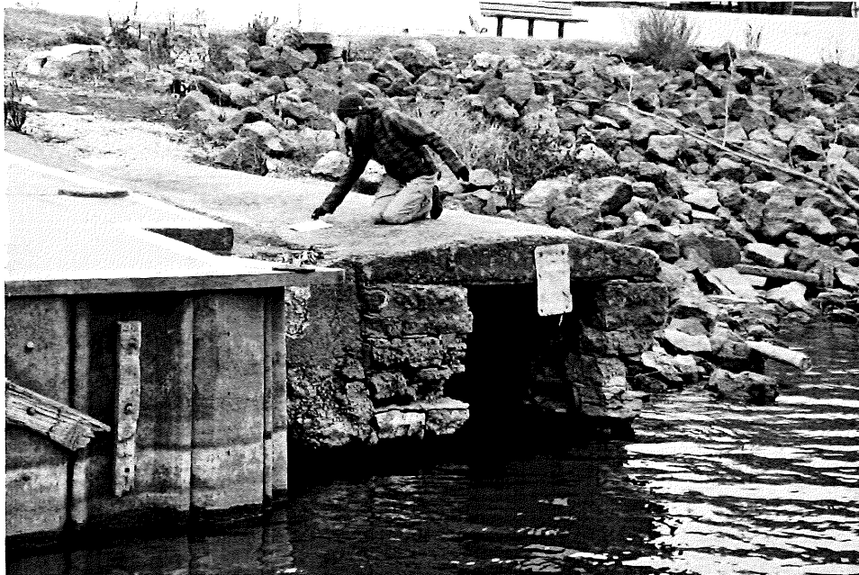
Fig. 252. Mississippi River. Red Wing Harbor and Levee, mortared limestone storm sewer outlet at the east end of the First Small Boat Harbor (facing S)
