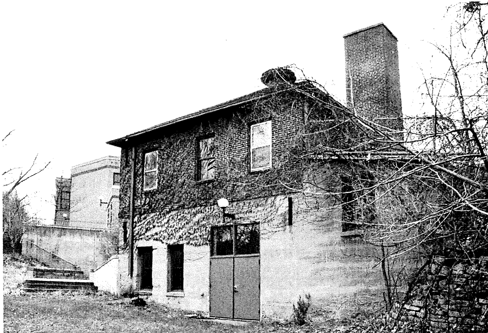
Fig. 337. 1166 Oak St. RW City Hospital & Old People's Home, east (rear) facade with poured concrete coal bin at right (facing SW)
