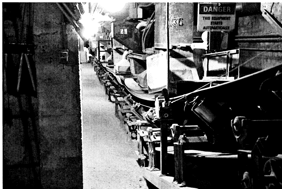
Fig. 205. 810 Levee Rd. Burdick Grain Co. Terminal Elevator, horizontal belt conveyor in the tunnel beneath the "6-pack" bank of bins west of the headhouse (facing W)
