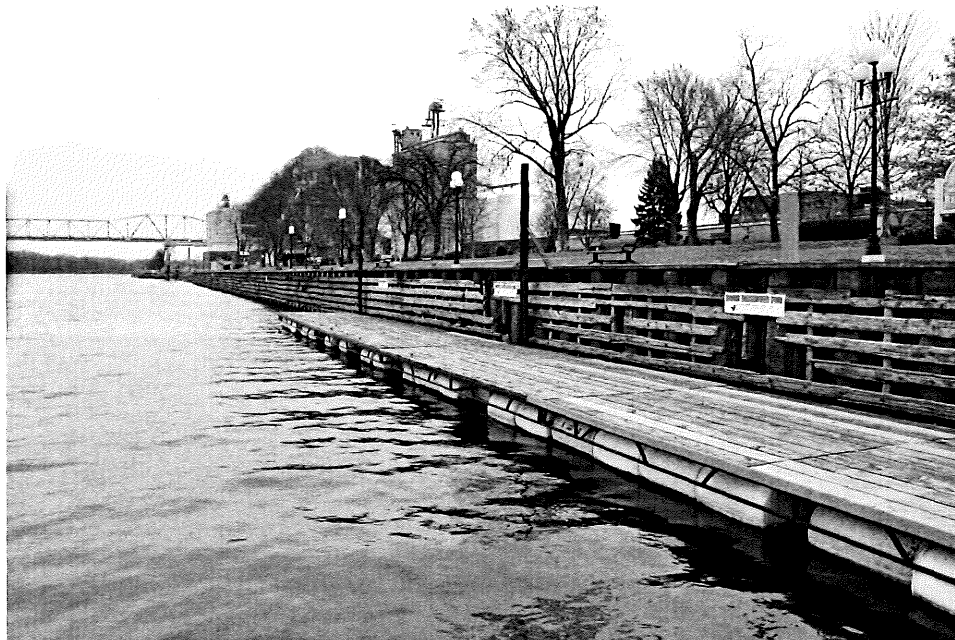
Fig. 253. Mississippi River. Red Wing Harbor and Levee, 600'-long Levee dock with timber fenders; Levee Park above (facing S)
