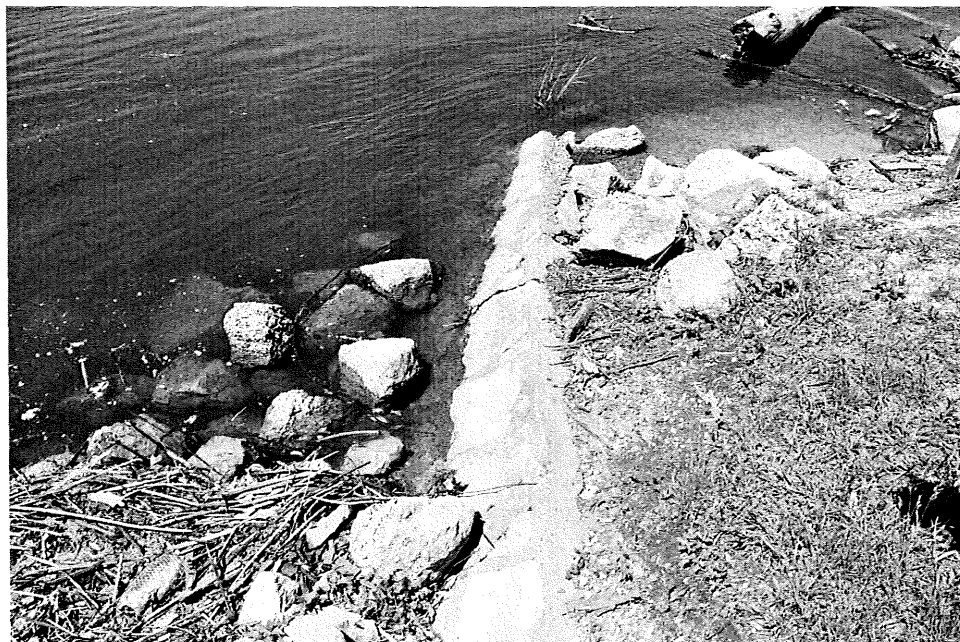
Fig. 251. Mississippi River. Red Wing Harbor and Levee, mortared stone wall remnant near the east end of the First Small Boat Harbor (facing NE)
