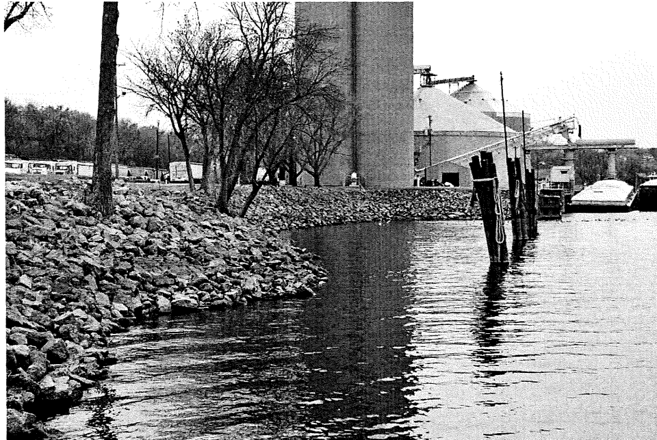
Fig. 250. Mississippi River. Red Wing Harbor and Levee, grain barge mooring dolphins and riprapped bank at the First Small Boat Harbor between Burdick Grain and Broad Street (facing SW)
