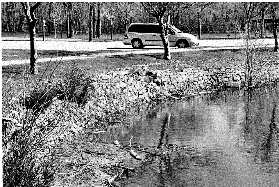
Fig. 247. Mississippi River. Red Wing Harbor and Levee, retaining wall of dry laid salvaged concrete (ca. 1956) on the north edge of the Lower Harbor (facing N)
