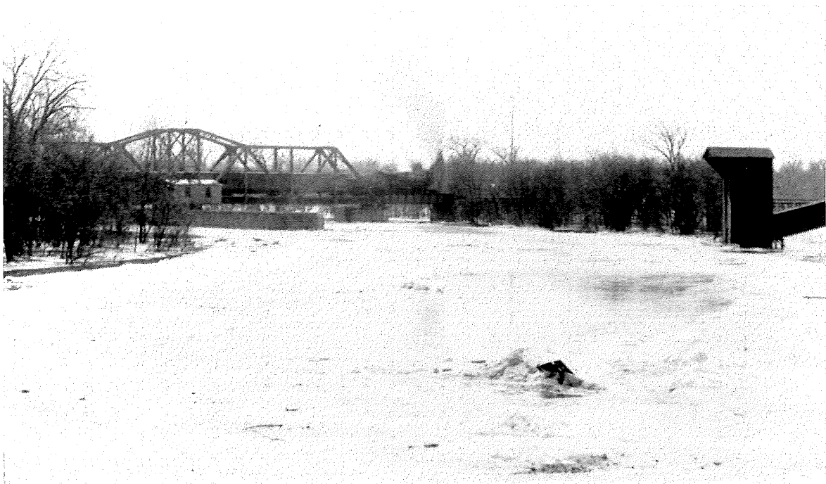
Fig. 20. April 1916 photo of the Soo Line Swing Bridge, the Red River Transportation Company Elevator, and the river as the ice is melting in a high-water spring; note the swing bridge's timber draw rest (over which the span opens) that projects from the central bridge pier; facing southwest, taken April 17, 1916 (Pennington County Historical Society)
