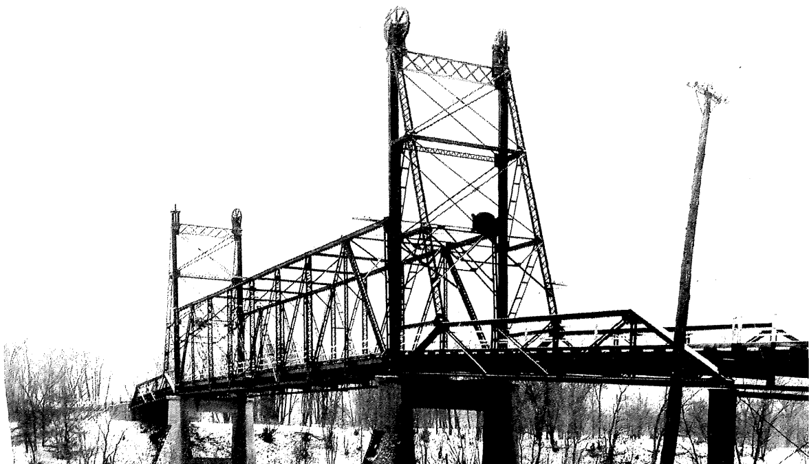
Fig. 22. The 1913 road bridge after its lift-bridge counterweights had been removed in 1932; wooded North Dakota bank of the river; facing northwest, ca. 1940 (Mn/DOT photo)
