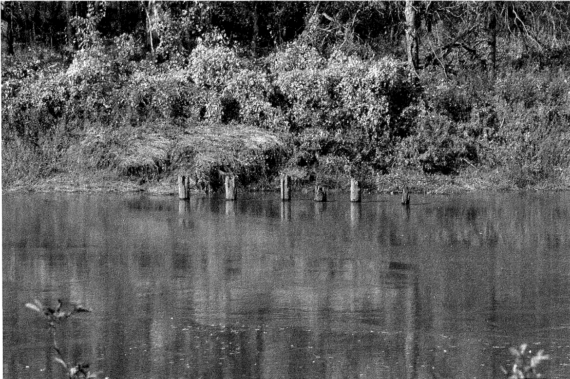
Fig. 29. Another view of the pilings from the Red River Transportation Company Elevator; the water was high when this photo was taken and a local resident said the piers usually project farther out of the water; facing northwest, 2010 (Gemini Research photo)
