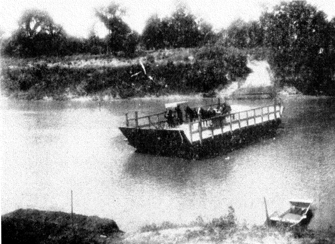
Fig. 19. Ca. 1910 photo of the Oslo Ferry; the Oslo ferry landing and a rowboat are in the foreground; the North Dakota ferry landing is across the river; the ferryman is beneath a sun canopy next to a windlass; right of the operator is a wagon pulled by two horses; there is probably another person left of the ferryman; facing northwest ( Oslo Golden Jubilee 1955: 74)
