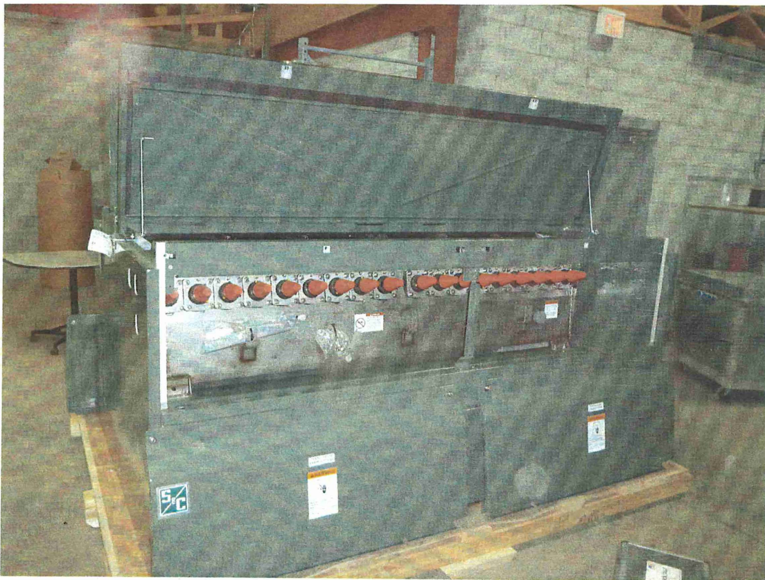
Image 1 – S&C Vista Model 624 DSG (termination side, enclosure open)
