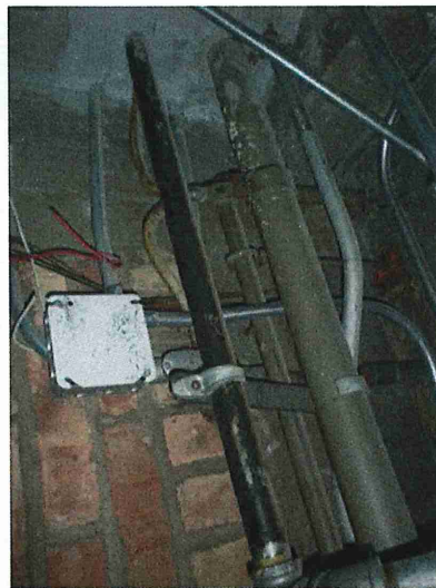
Photo 9: Unit 4 ground tied to pipe
