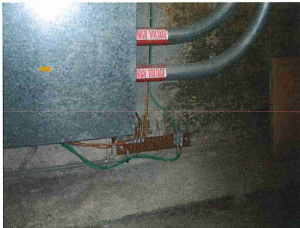
Photo 16: Power Plant Ground bus
