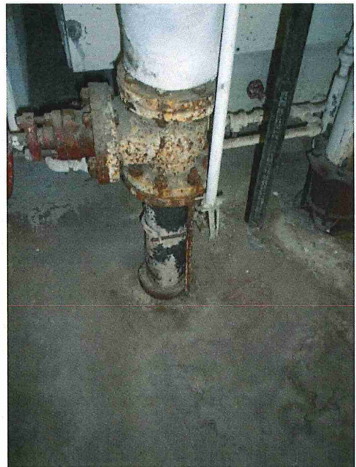
Photo 17: Power Plant Water service connection
