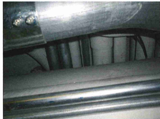
Photo 4: Bldg. 60 ground wire tied to water pipe
