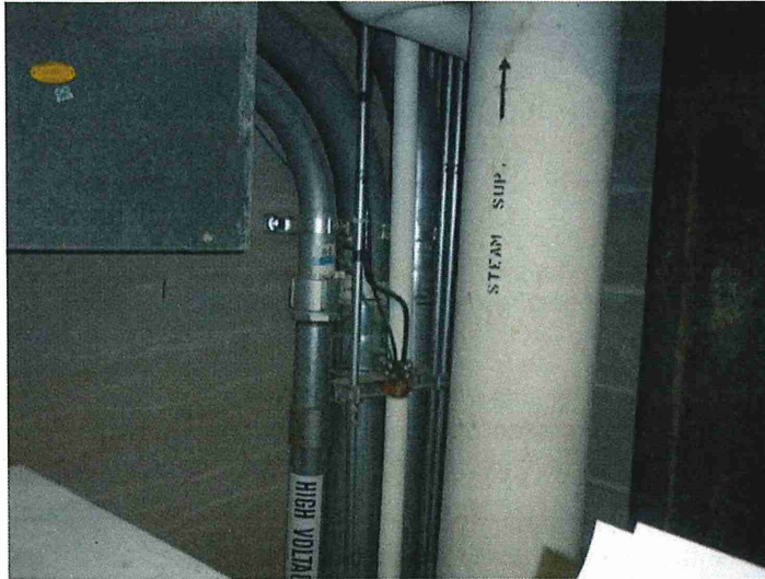
Photo 15: Gym Grounds tied together at water pipe
