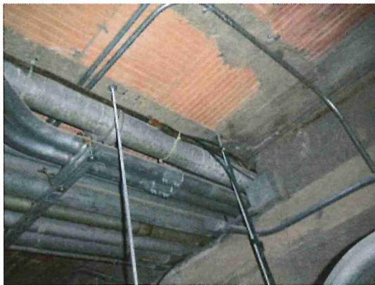
Photo 3: Bldg. 60 ground wires tied together
