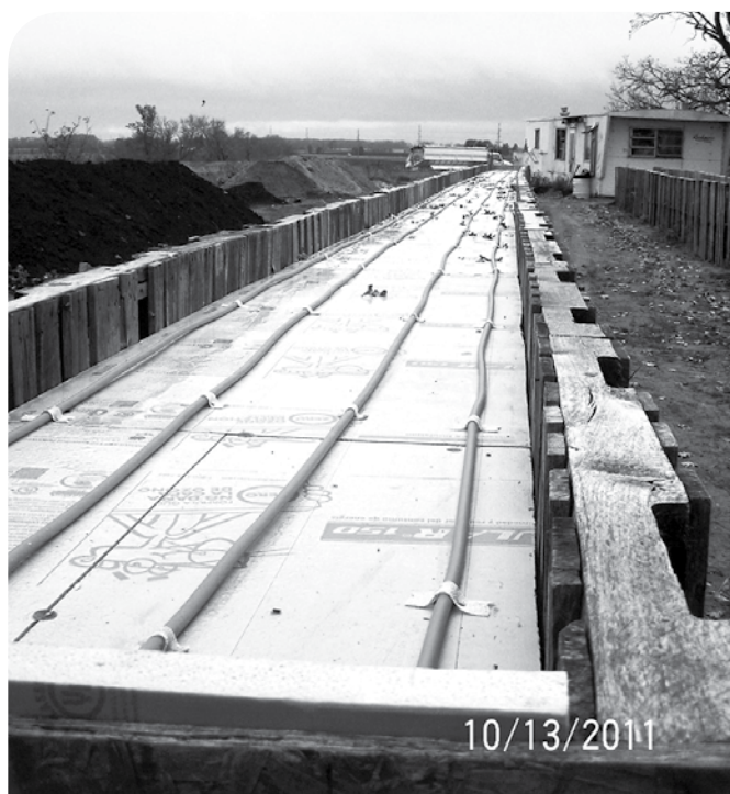
View of the X-beds facing south before filling beds with soil, with the Pex-al-Pex tubing. The soil we used to fill the beds is in piles on the left.
