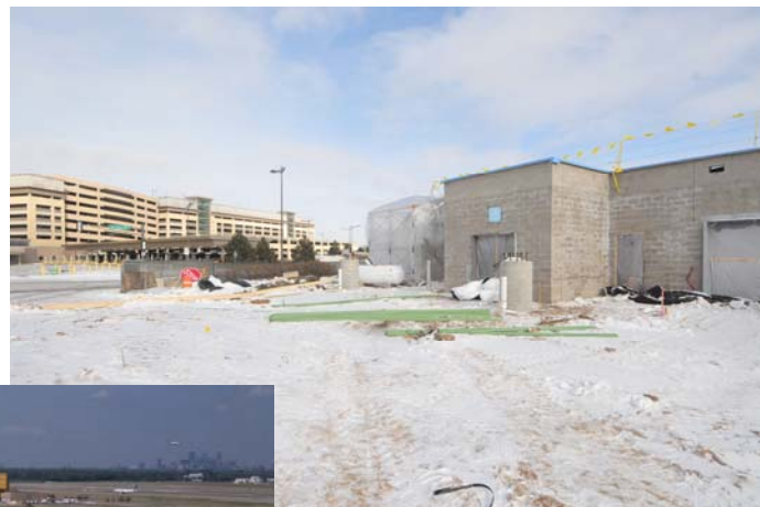
Building shell construction that will house the new baggage handling/inspection system at T-2
