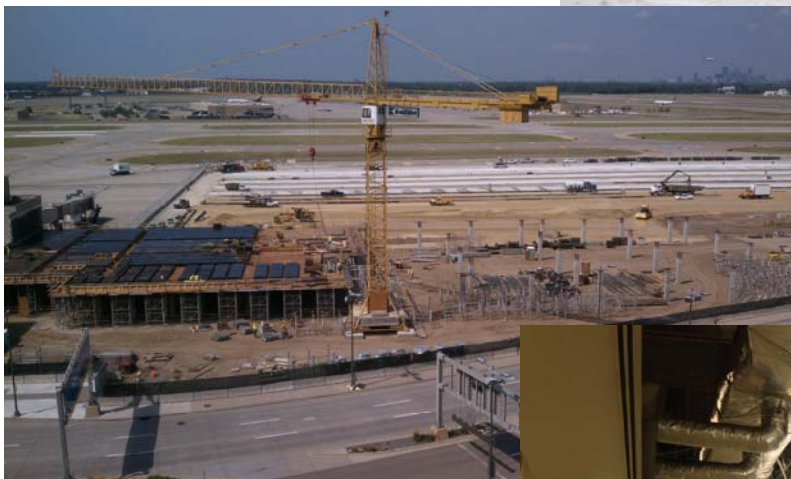
Building shell construction that will house the new baggage handling/inspection system at T-2
