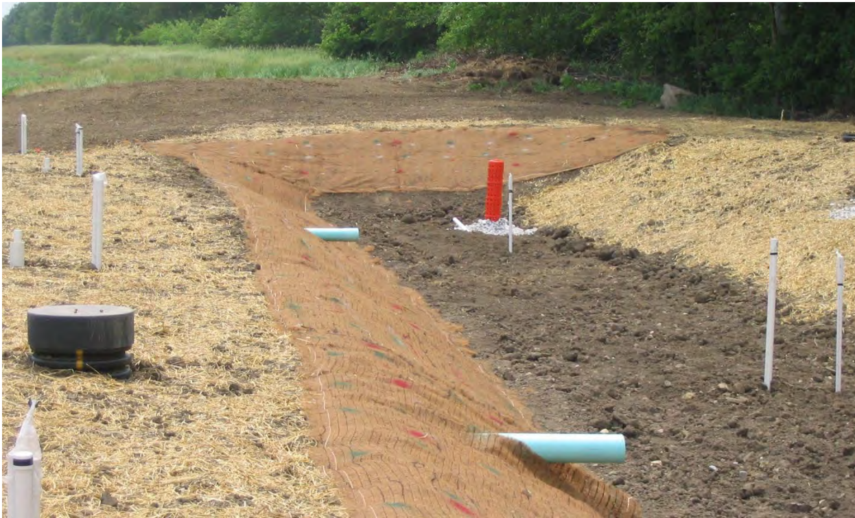
Constructed Wetland under Construction
