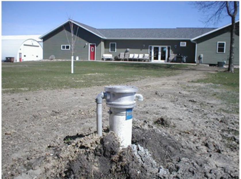
*New private wells that are properly constructed, such as this one, can help to protect groundwater sources from contamination, such as nitrates. This well still needs to have finished landscaping.*
