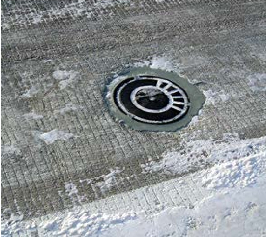
Spray head in bridge deck
