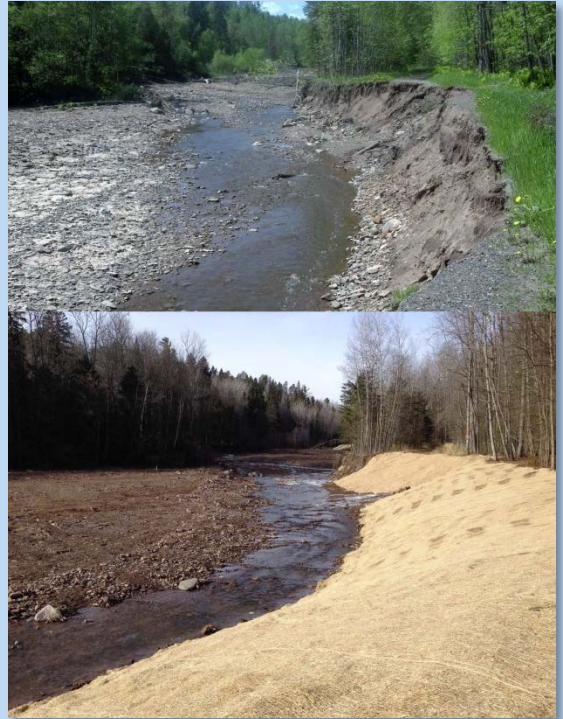
Duluth’s Mission Creek, before and after stabilization work.
