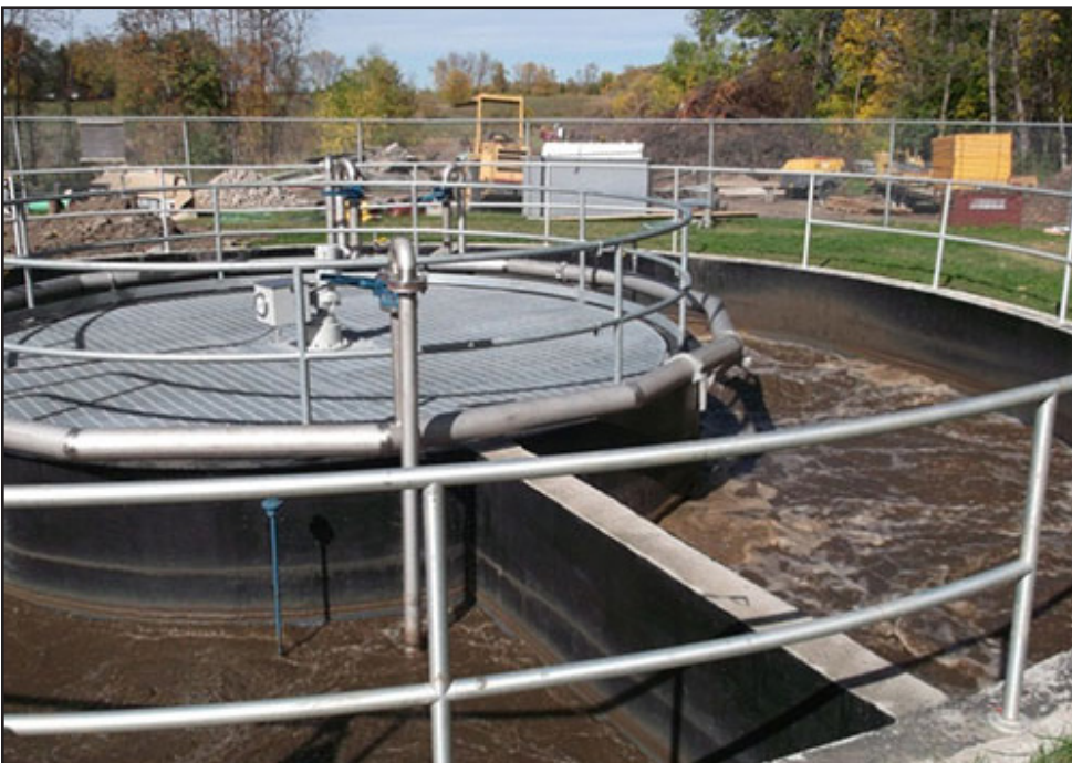
New treatment facility.
