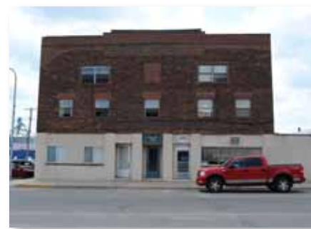
Potential multi-family rehabilitation project in Clara City.
