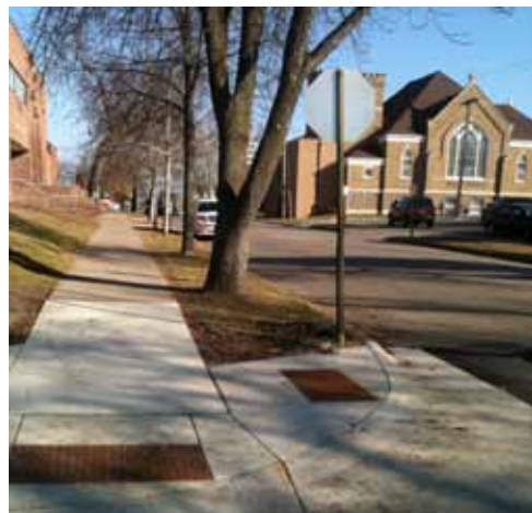
Newly constructed curb ramps in Dawson
