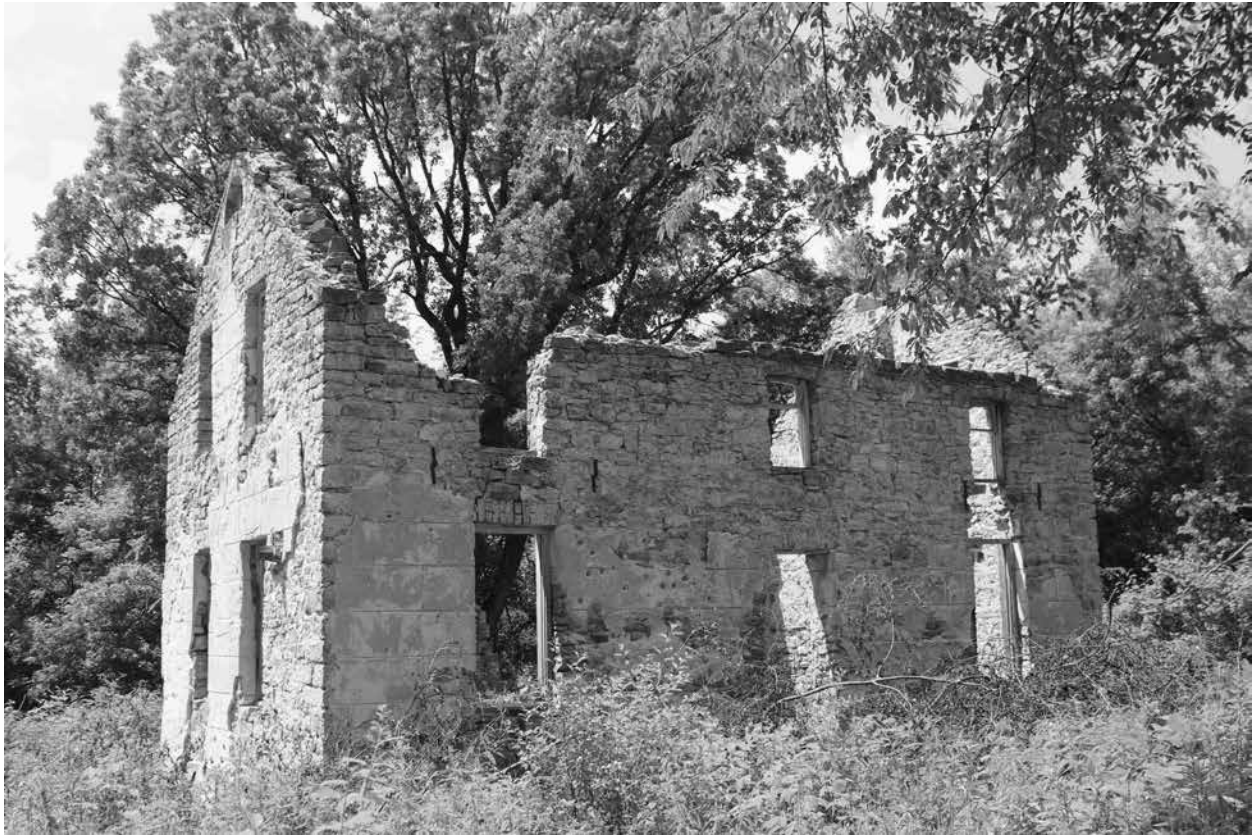
Cordes House ruins in Goodhue County.
