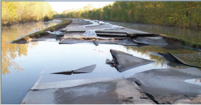
Water covers a flood-damaged section of Hwy 169 a few miles north of St. Peter. Photo by Thomas Zimmerman
