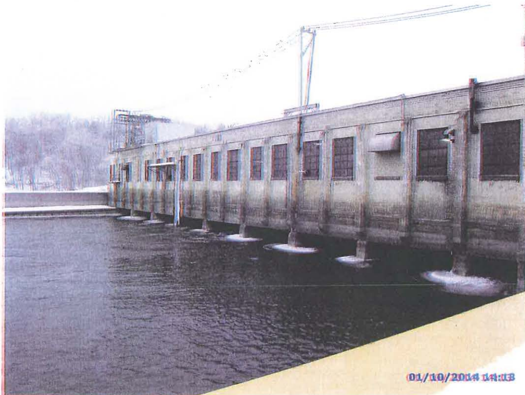
Downstream side of powerhouse (looking west)
