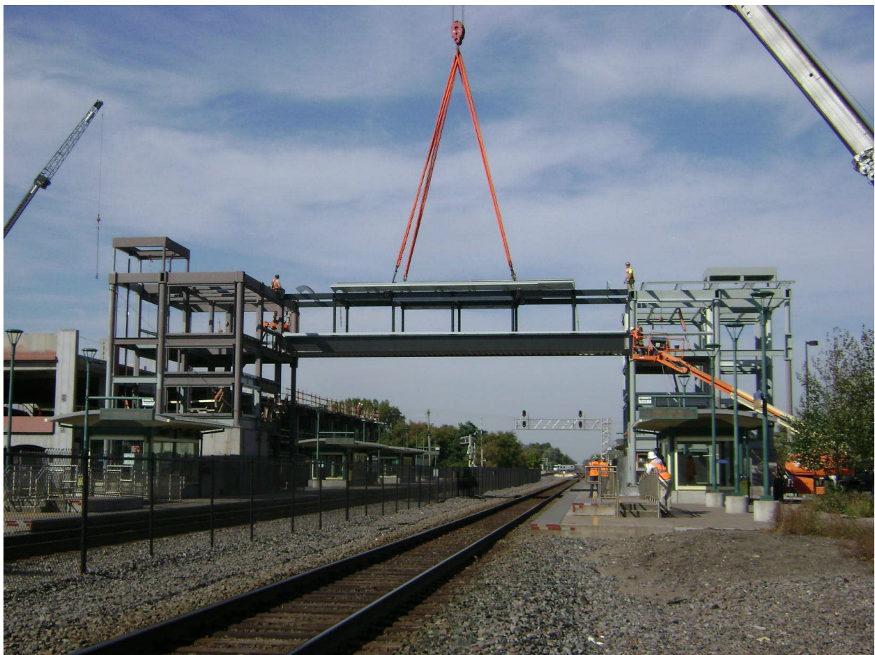
Figure 11: Installation of the pedestrian bridge, October 2013
