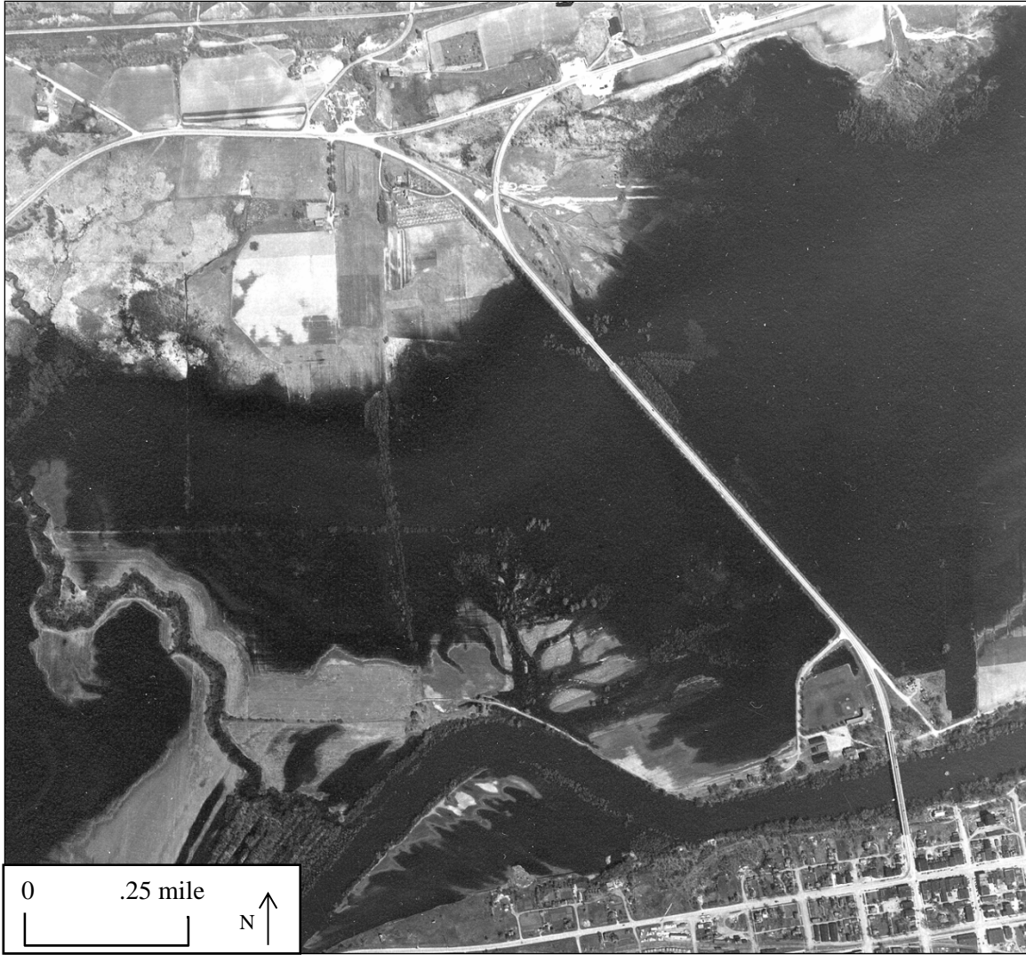
Figure 7. 1947 Aerial Photograph of Project Area During High Water Period.
