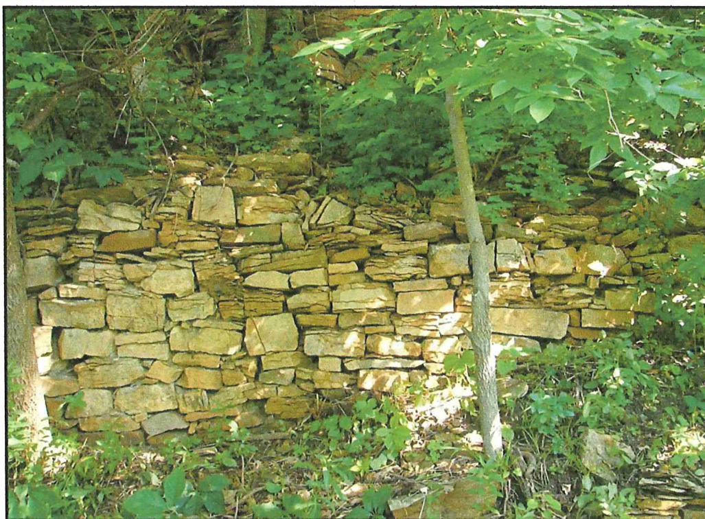
FIGURE 21. TALLEST SEGMENT OF RETAINING WALL, VIEW TO NORTHWEST
