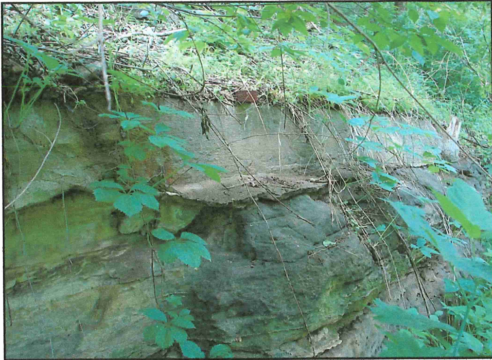
FIGURE 26. CONCRETE FACING ABOVE CAVE 2, VIEW TO NORTH
