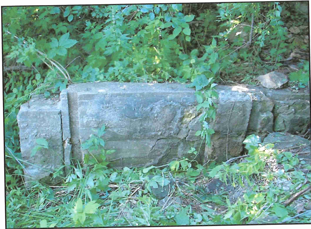
FIGURE 24. CONCRETE ADDITION TO WEST OF CAVE 1 MOUTH, VIEW TO WEST
