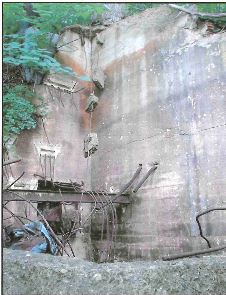
FIGURE 16. REMAINS OF ST. PETER STATE HOSPITAL PUMP HOUSE
